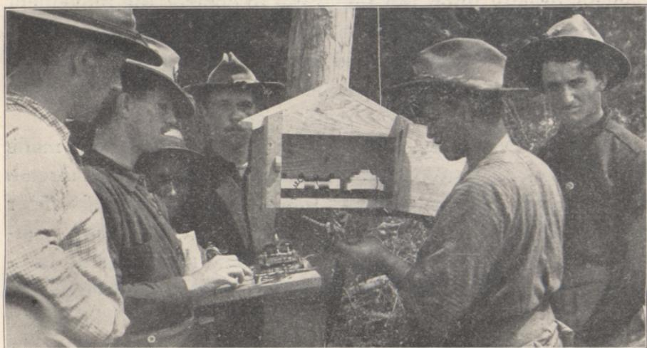
PLATE II. TESTING SUBMARINE CABLE, SHOWING CABLE BOX ARRANGEMENTS.
