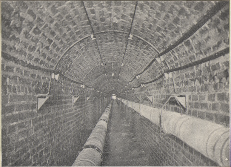
PLATE II. IN TUNNEL, LOOKING SOUTH TOWARD POWER HOUSE.
