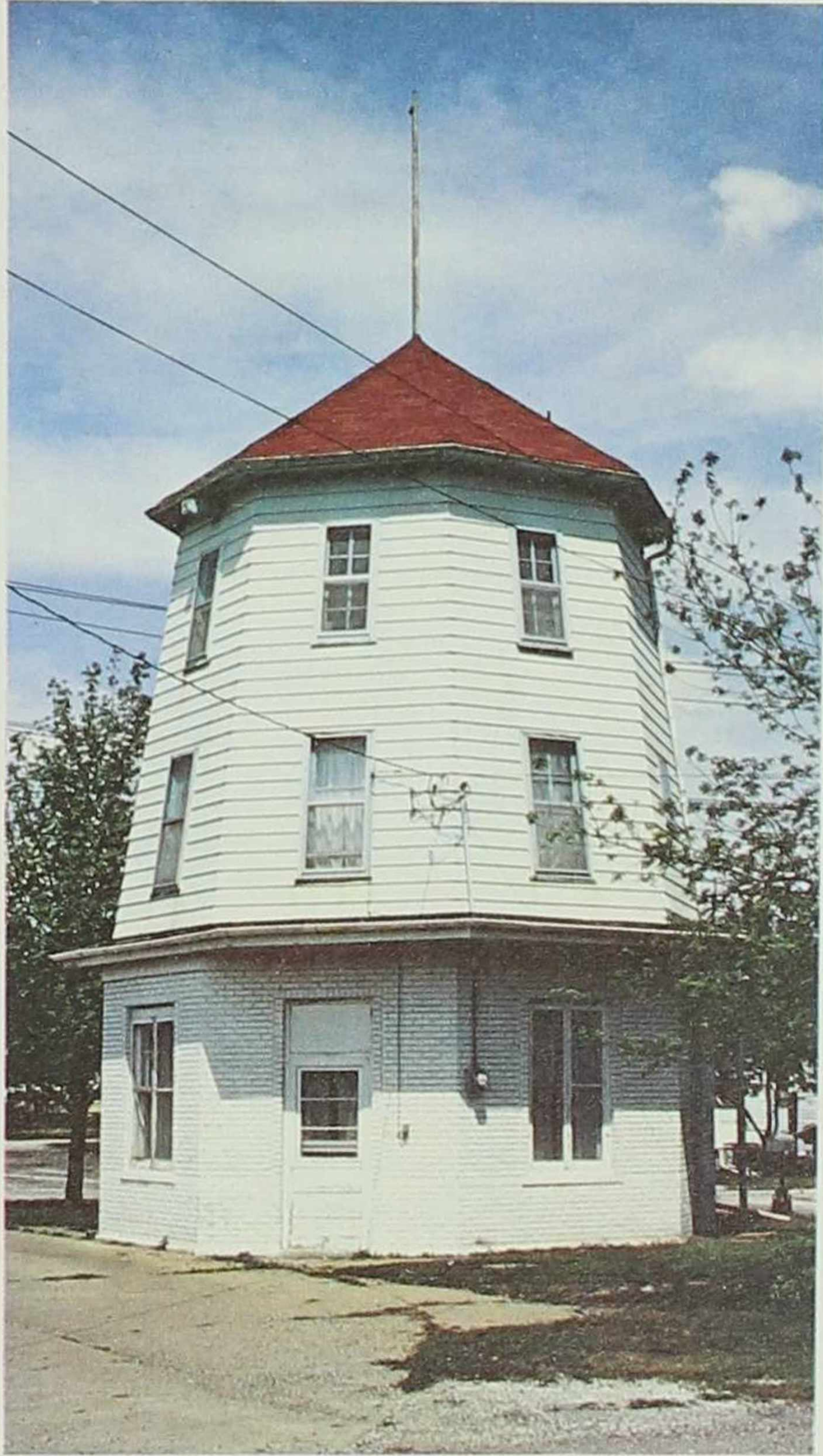
The Mill as it appears today, considerably altered from its original form. Aluminum siding has been installed over the original stucco on the second and third floors and the arms and railings have been removed (courtesy of the author).
