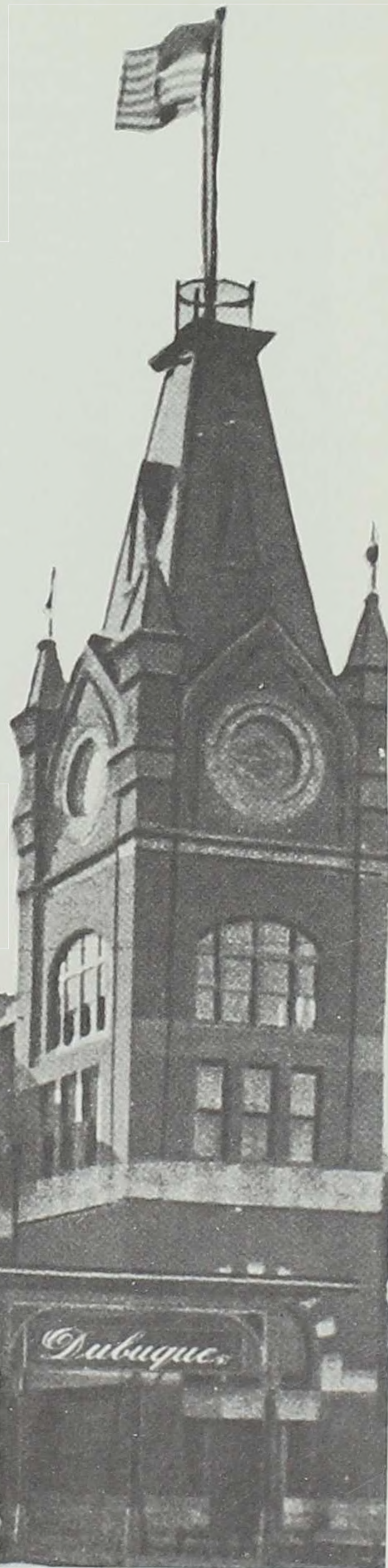
The Illinois Central built this large brick station in Dubuque in 1887. The building measured 290 feet long by 50 feet wide and was modernized by the railroad during World War II. The decorative tower reflects Eastern styles.
