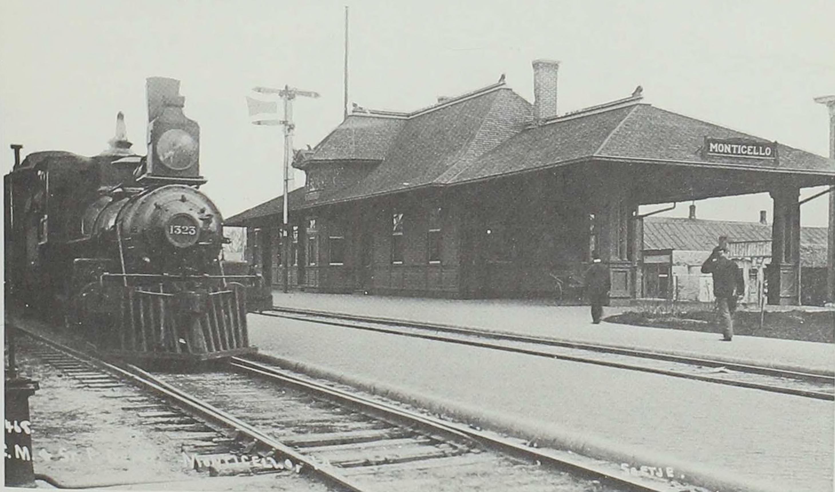
Dating from 1905, the Monticello, Iowa station is of a design often used for county-seat communities. Situated at the junction of two Milwaukee Road branches, the structure has a typical carriage canopy.
