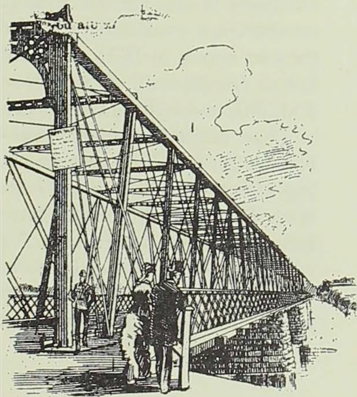
Court Avenue Bridge over the Des Moines.
