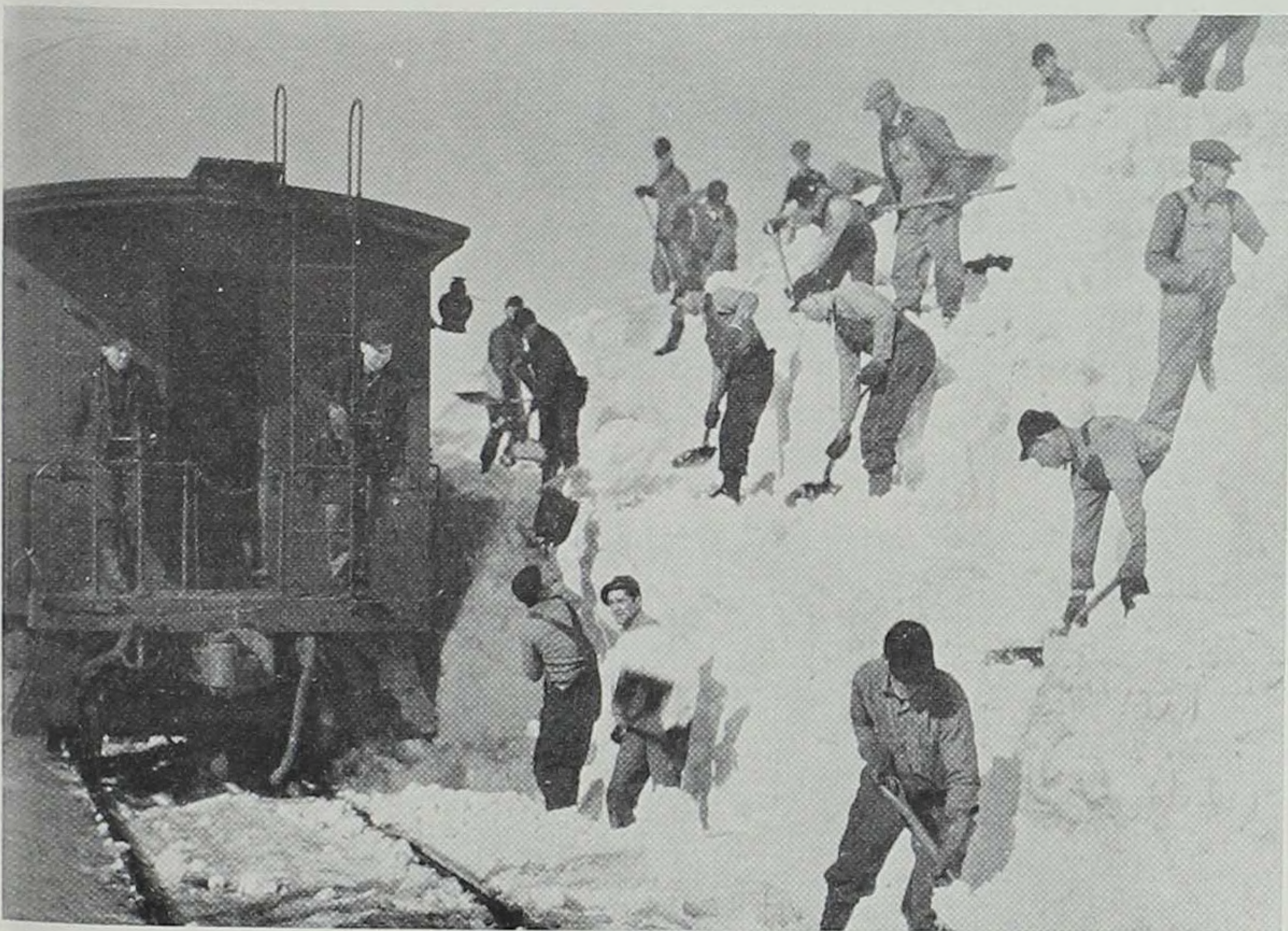
Trackmen digging out a marooned freight train during the winter of 1936. During this severe storm the Illinois Central sent snow-fighting equipment from all over its System to aid the hard-hit Iowa Division.
