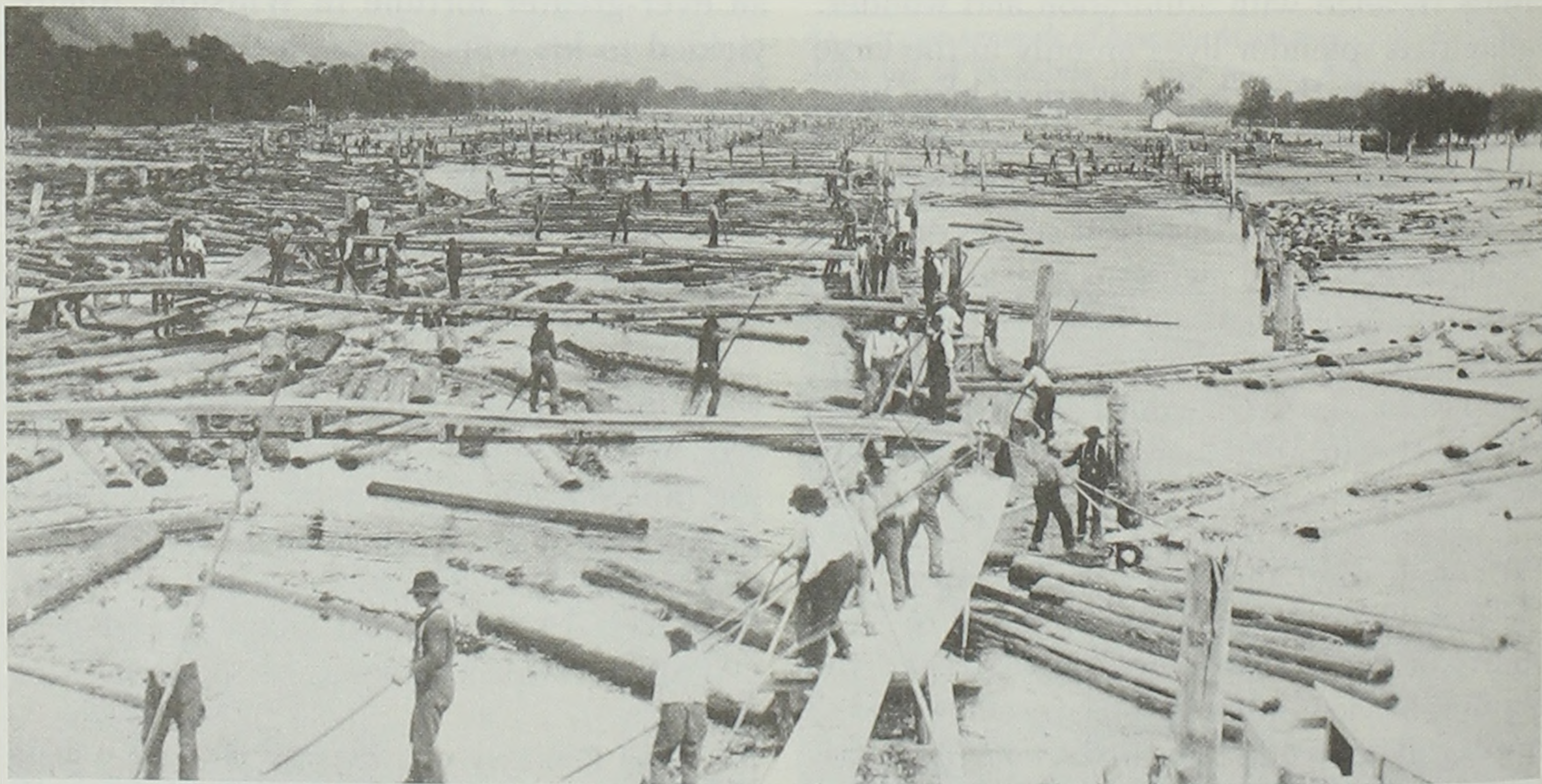
In backwater sloughs, surefooted raftsmen first chained the longest logs into loose frames, in which other logs would float. A raft often contained a million feet of logs, covering three acres. (SHSI)
