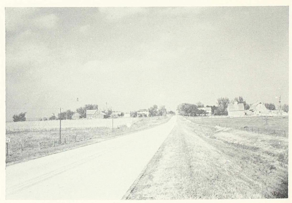
Typical of the paved roads built in the 1920's and early 1930's is this 18-foot highway near Guthrie Center. The paving cost about \$30,000 per mile.
