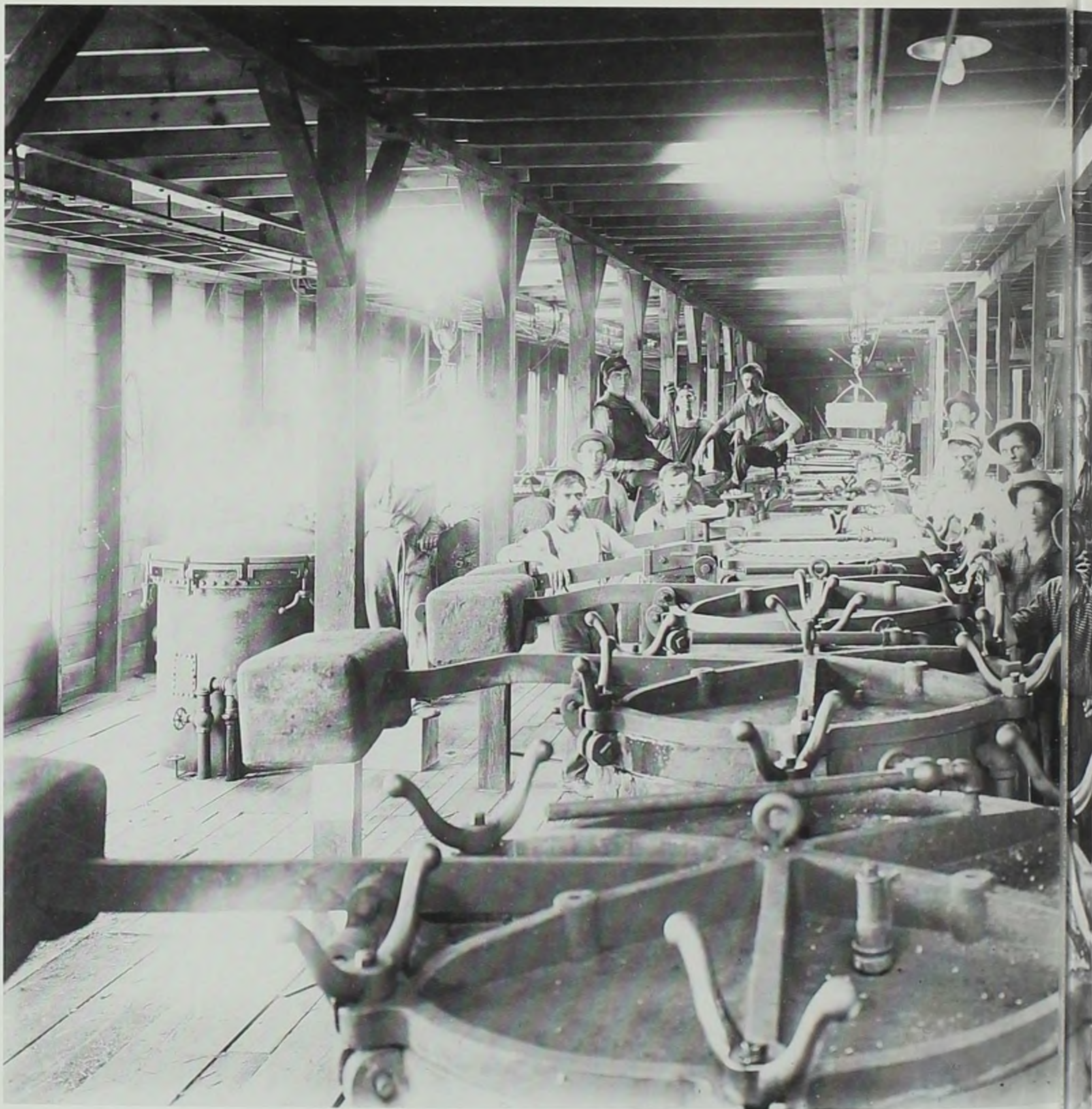
Left: Cans filled with produce are placed in enormous crate-like trays and then lowered into the retorts (above) for steam heating.
