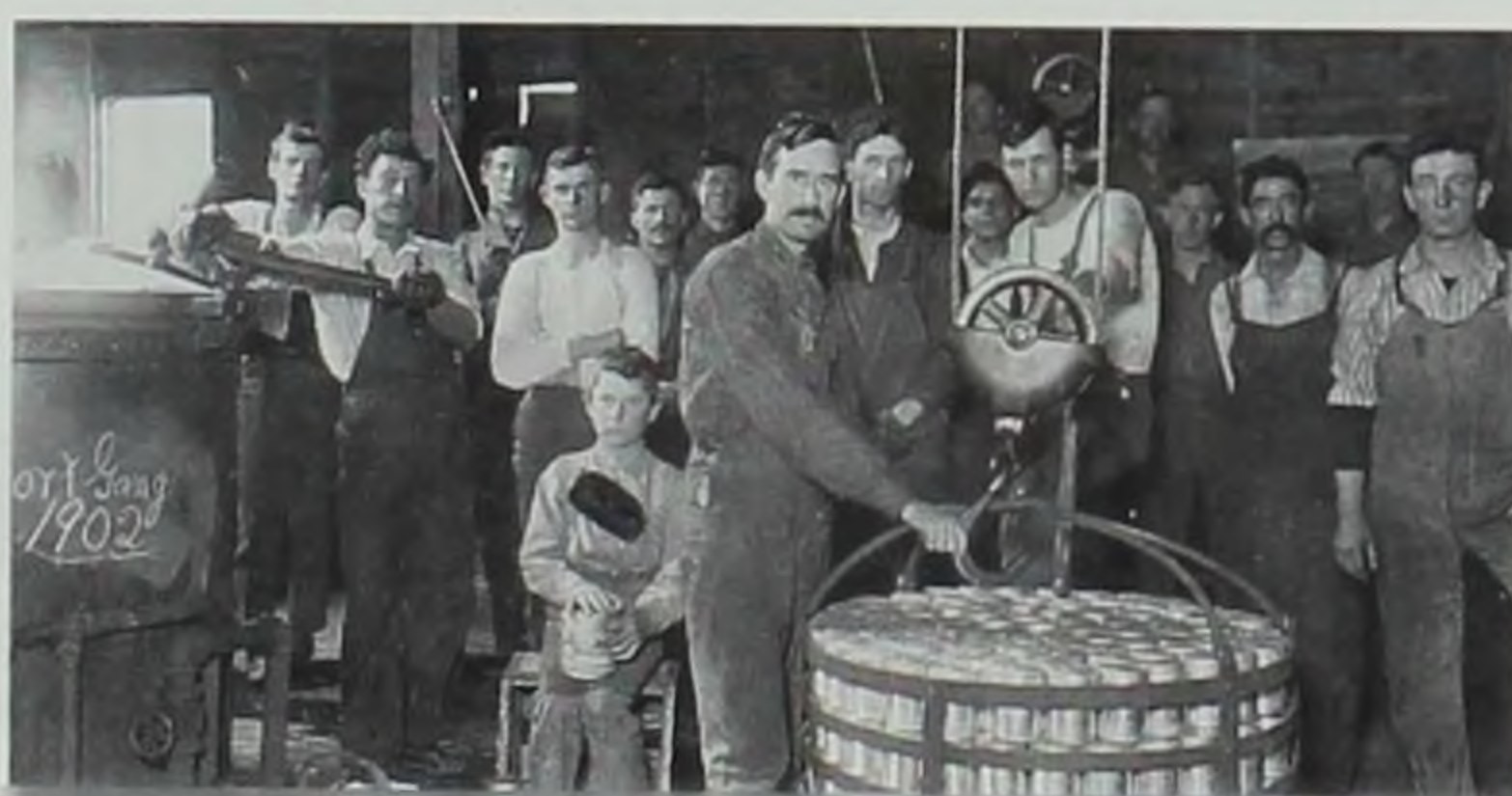
Left: Cans filled with produce are placed in enormous crate-like trays and then lowered into the retorts (above) for steam heating.
