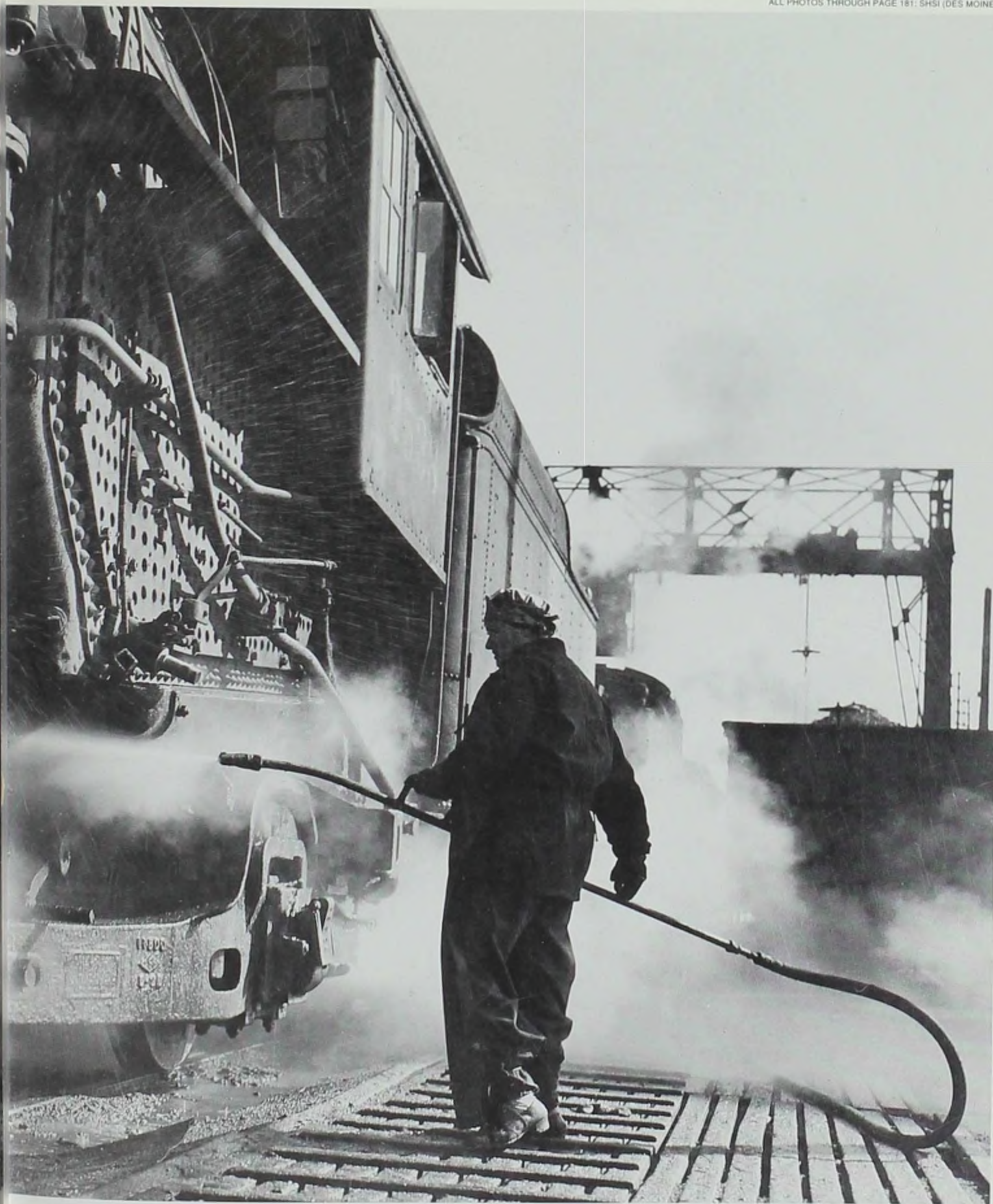
Marcella Kees, one of the Clinton WIPes, gives a locomotive a bath—a job, according to the Clinton Herald , “far different from the chore of washing out a few things at home.” In order to make women doing such heavy work seem “natural,” traditionally male jobs held by women were often described in feminized terms.
