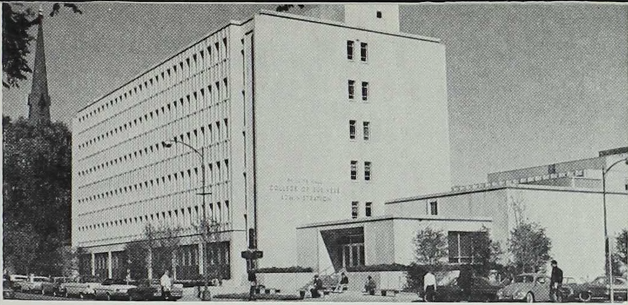
Phillips Hall, new home of the College of Business Administration.
