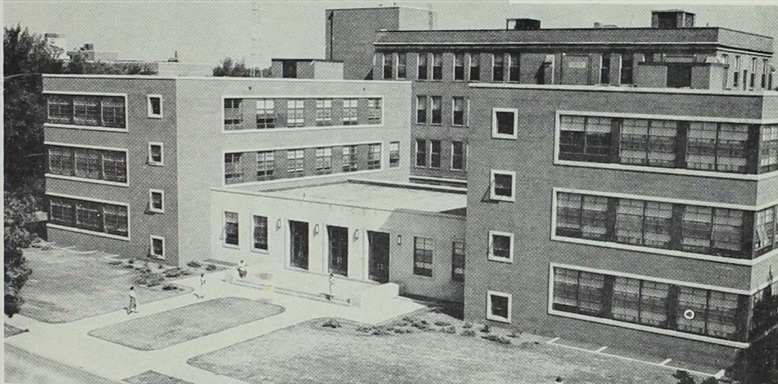
The addition to the Science Building, finished in 1955.
