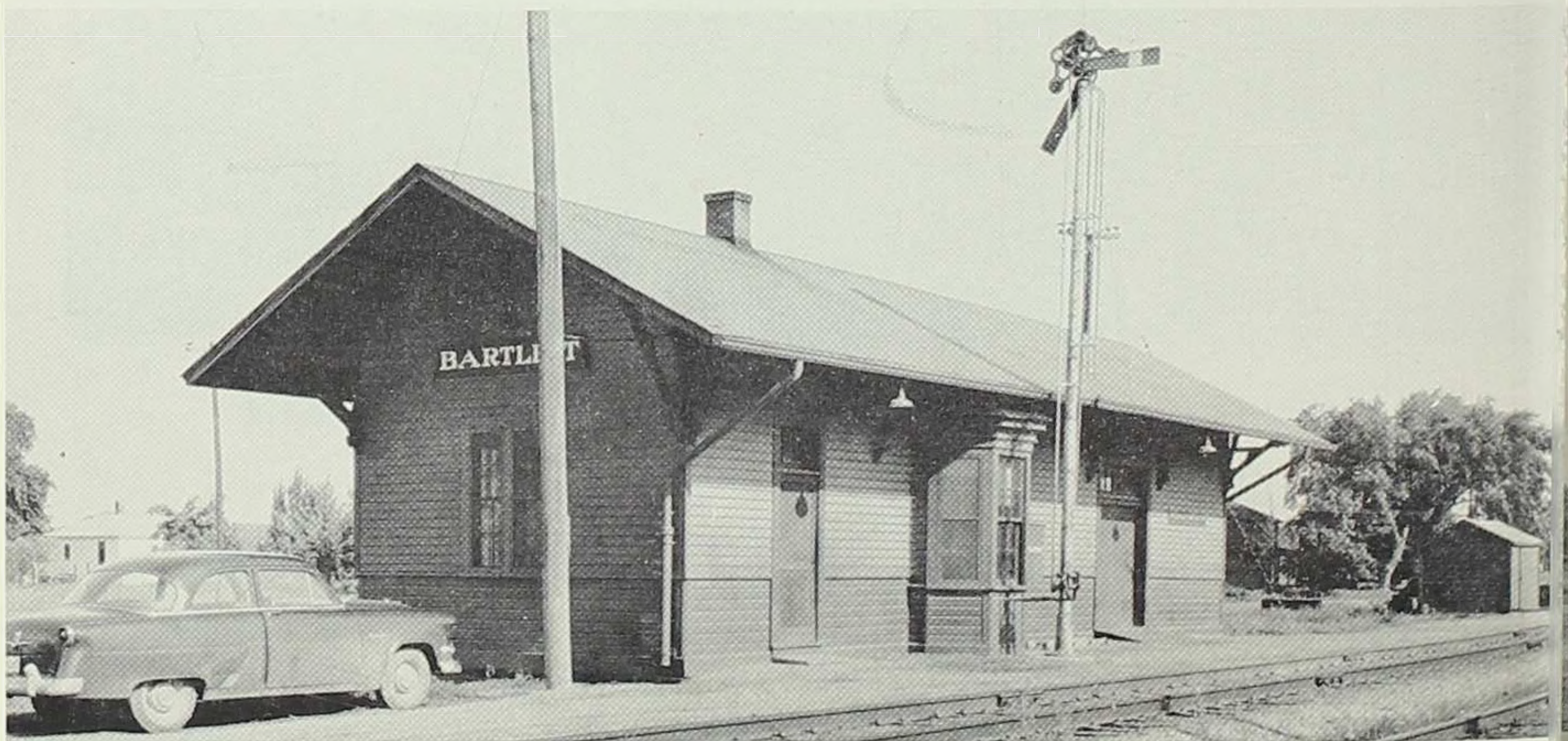
Bartlett railroad station on Burlington "high iron" between Council Bluffs and Kansas City.
