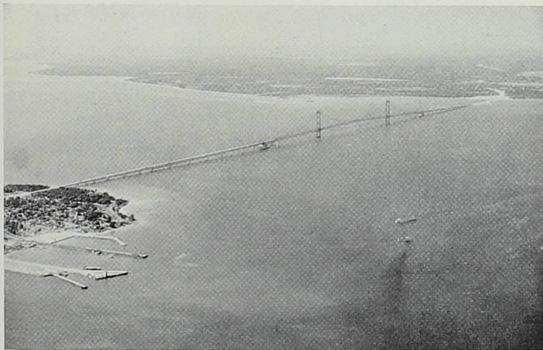
New Bridge opened in 1958 across Straits of Mackinac to St. Ignace. It was along the north shore of Lake Michigan that Joliet and Marquette paddled on their way to discover Iowa.
