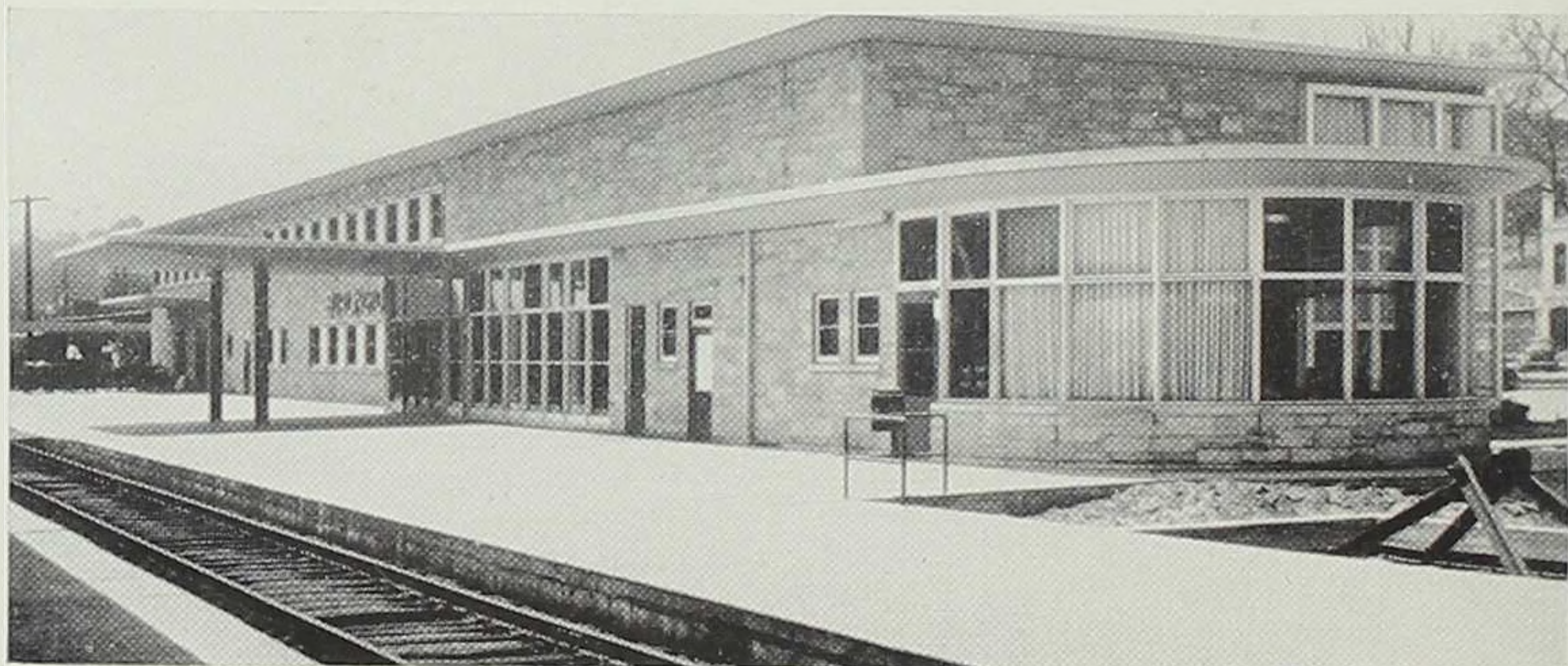
New Burlington Station at Burlington, Iowa
