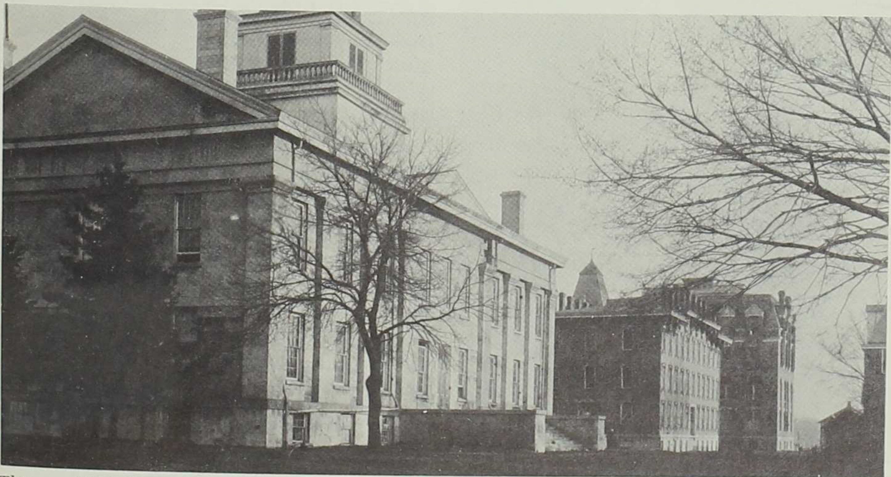
This pre-1901 photo shows clearly the recesses just below the roof and the platform intended for a west portico. The original plan evidently called for a portico, but it was not completed. The west portico was added during the 1920s. (courtesy of The University of Iowa)
