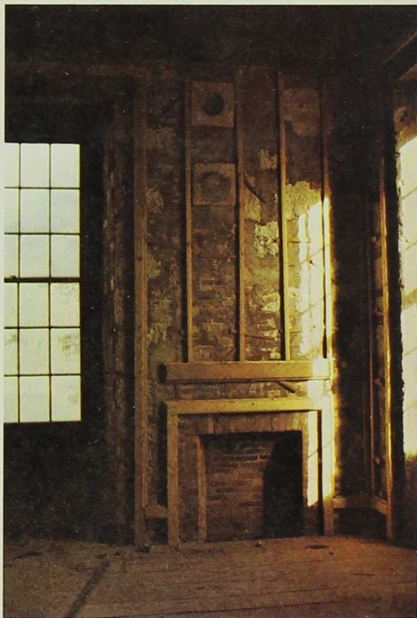
The walls of the Supreme Court Chamber, stripped of plaster, revealed the bricked-over fireplace and stovepipe holes. (courtesy of The University of Iowa, Don Roberts photo)
