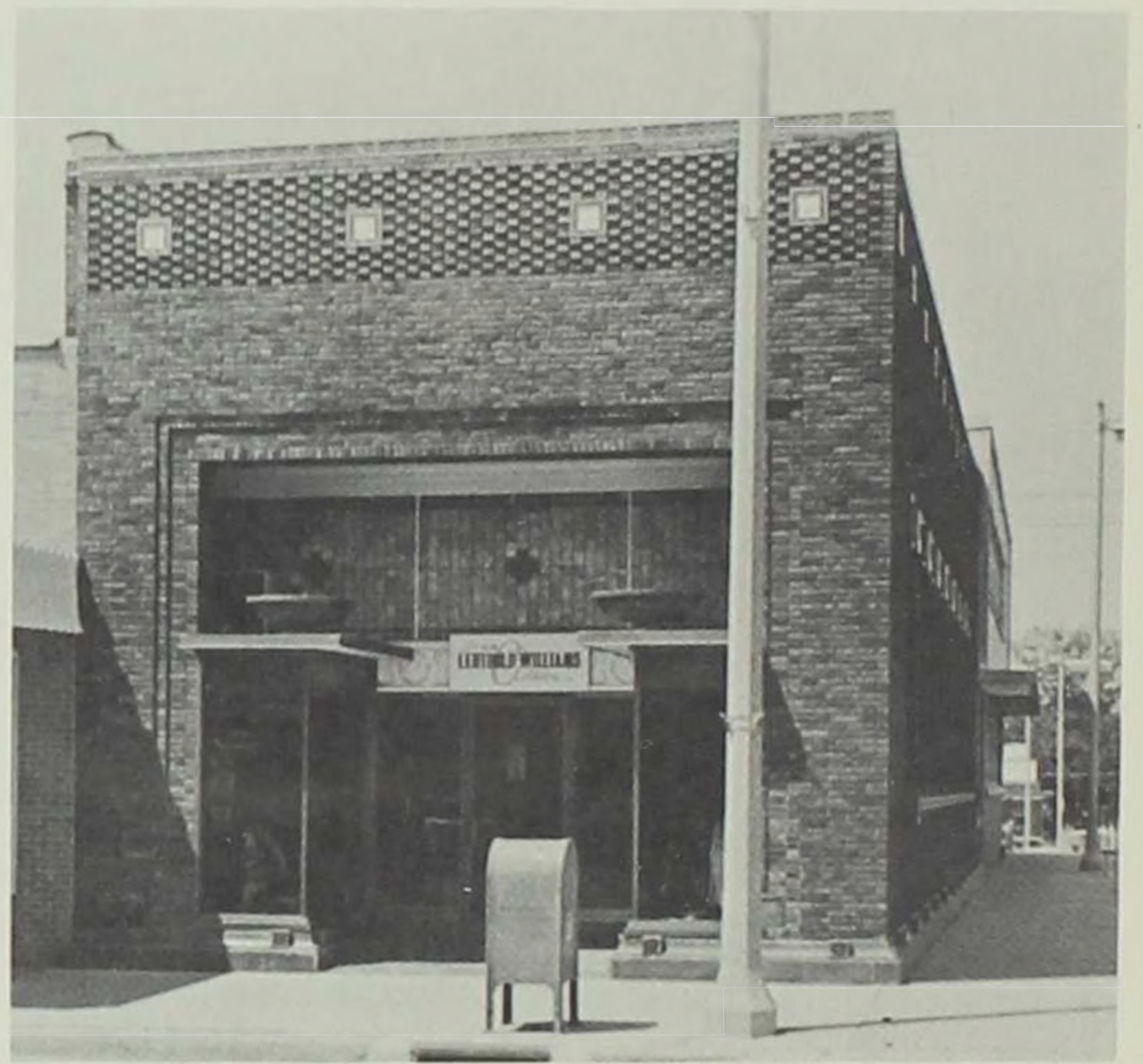
The Henry C. Adams Building in Algona (below) is a simple rectangular block. Subtle variations in the pattern of bricks, terra cotta panels and mouldings, and leaded glass windows (above left) enhance the structure's sturdy exterior. Completed in 1913, the building served as a realtor's office for many years and now houses Leuthold-Williams Clothiers. In the early 1970s, the owners engaged Des Moines architect William Wagner to install show windows sympathetic to the design of the original entrance (above right).
