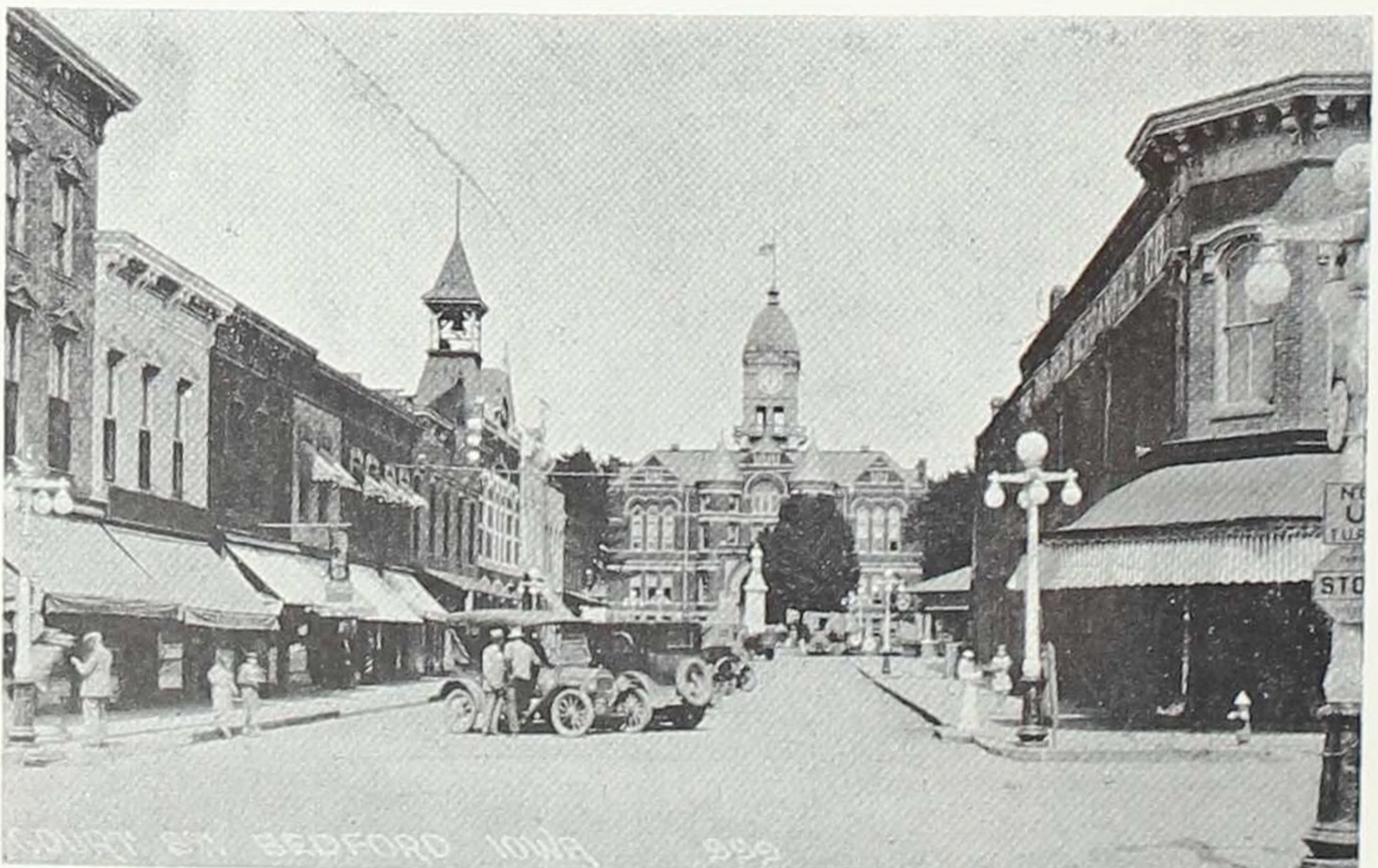
Court Street after paving. Five-cluster electric street lamp on corner. Third story of building on corner and City Hall cupola were later removed.
