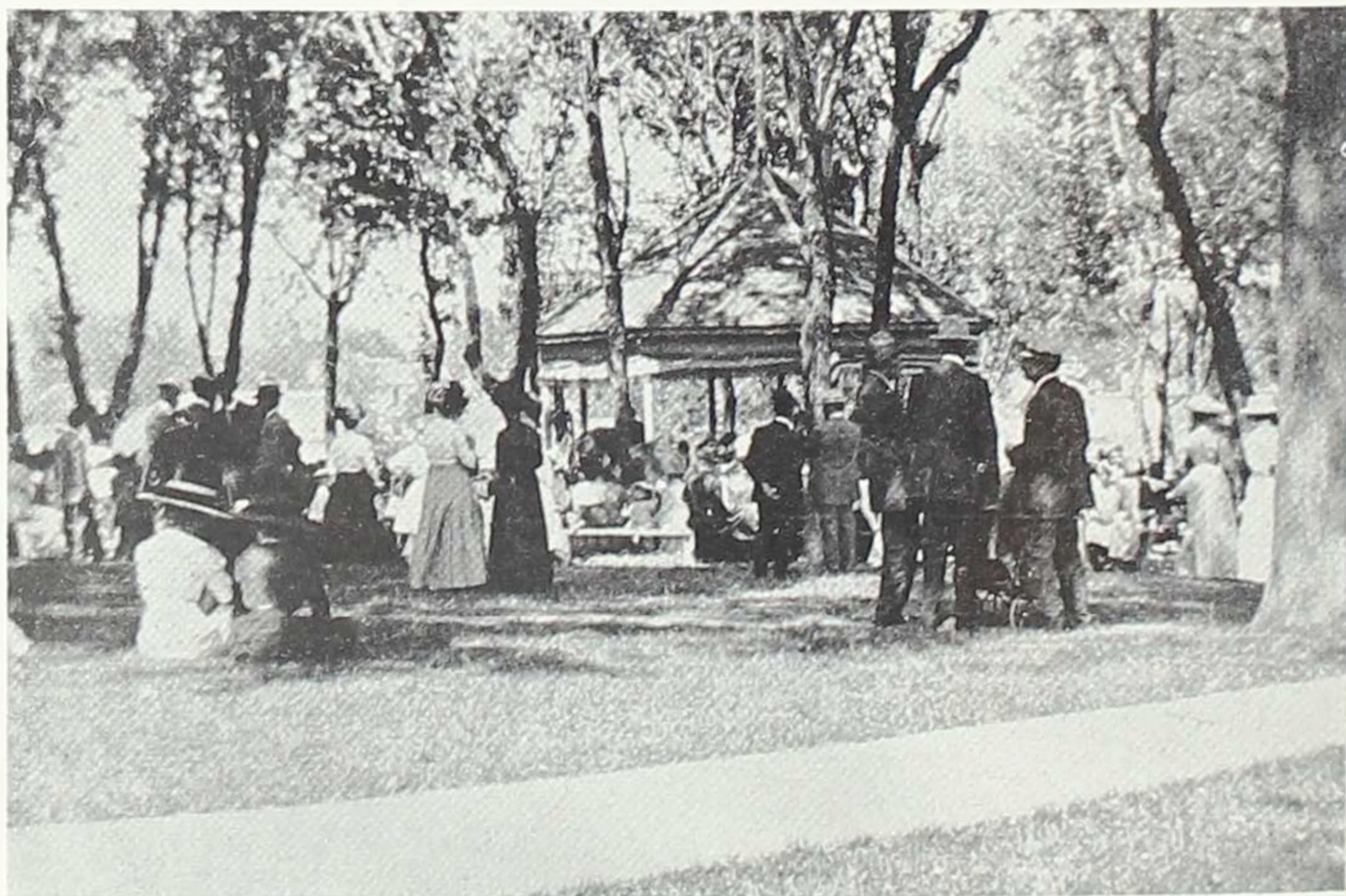
Bandstand in courtyard park. Formerly used for concerts, Memorial Day and Fourth of July addresses, and union church services in summer. Now dismantled.
