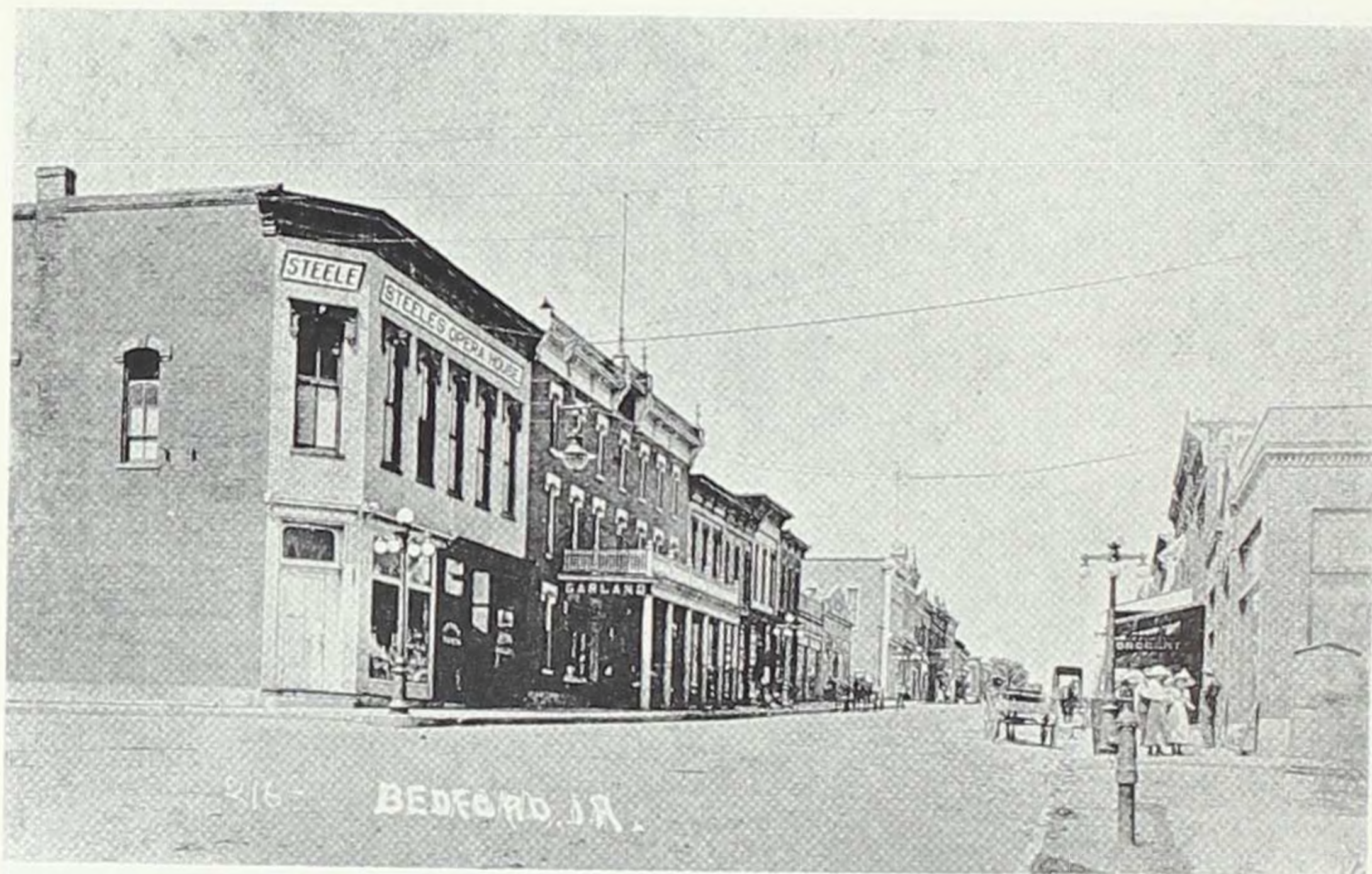
Steele's Opera House about 1905. Upstairs hall used for plays, dances, and meetings.
