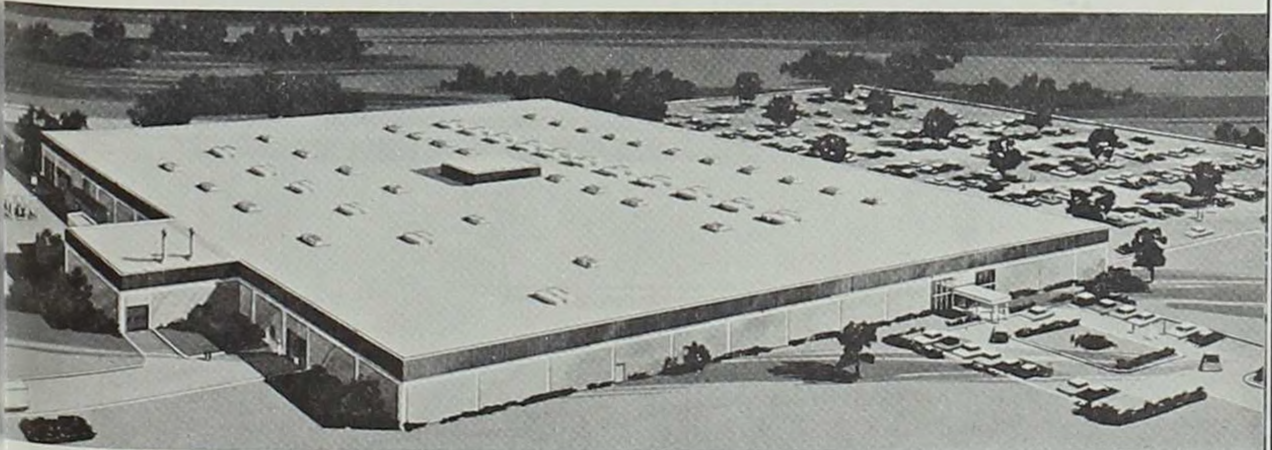
Fisher Governor Road plant
