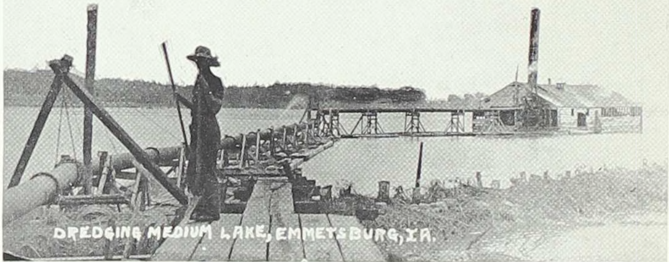
Steam dredge at work in 1913. Silt was pumped from the bottom of Medium Lake and forced through pipes onto the low ground lower right. Land was thus reclaimed for a park, boulevards, streets, and shoreline improvements.
