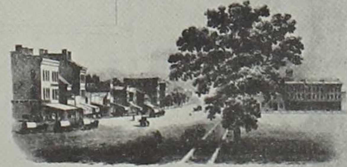
PART OF CLINTON STREET
