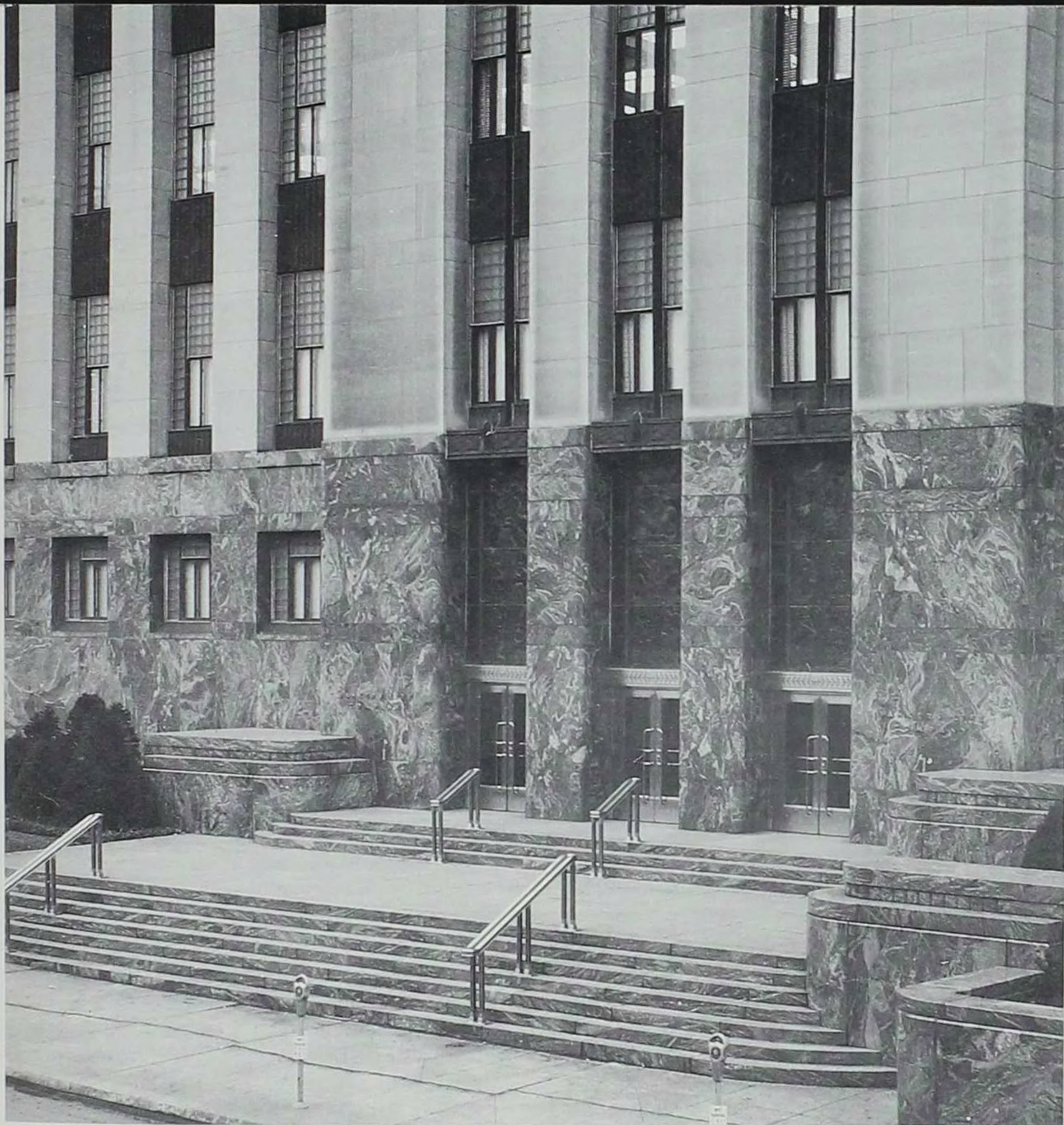
Rounded corners, strong lines, and rectilinear shapes mark the building. The three glass murals (over each door) are recessed in a sheathe of rainbow granite. A walkway has since been built over this entrance.
