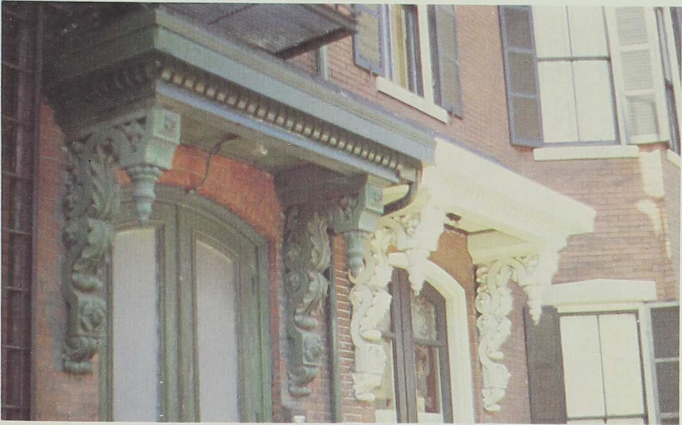
Painted to accentuate their rich design, these brackets from the 1892 catalogue grace a set of doorways in Springfield, Massachusetts.
