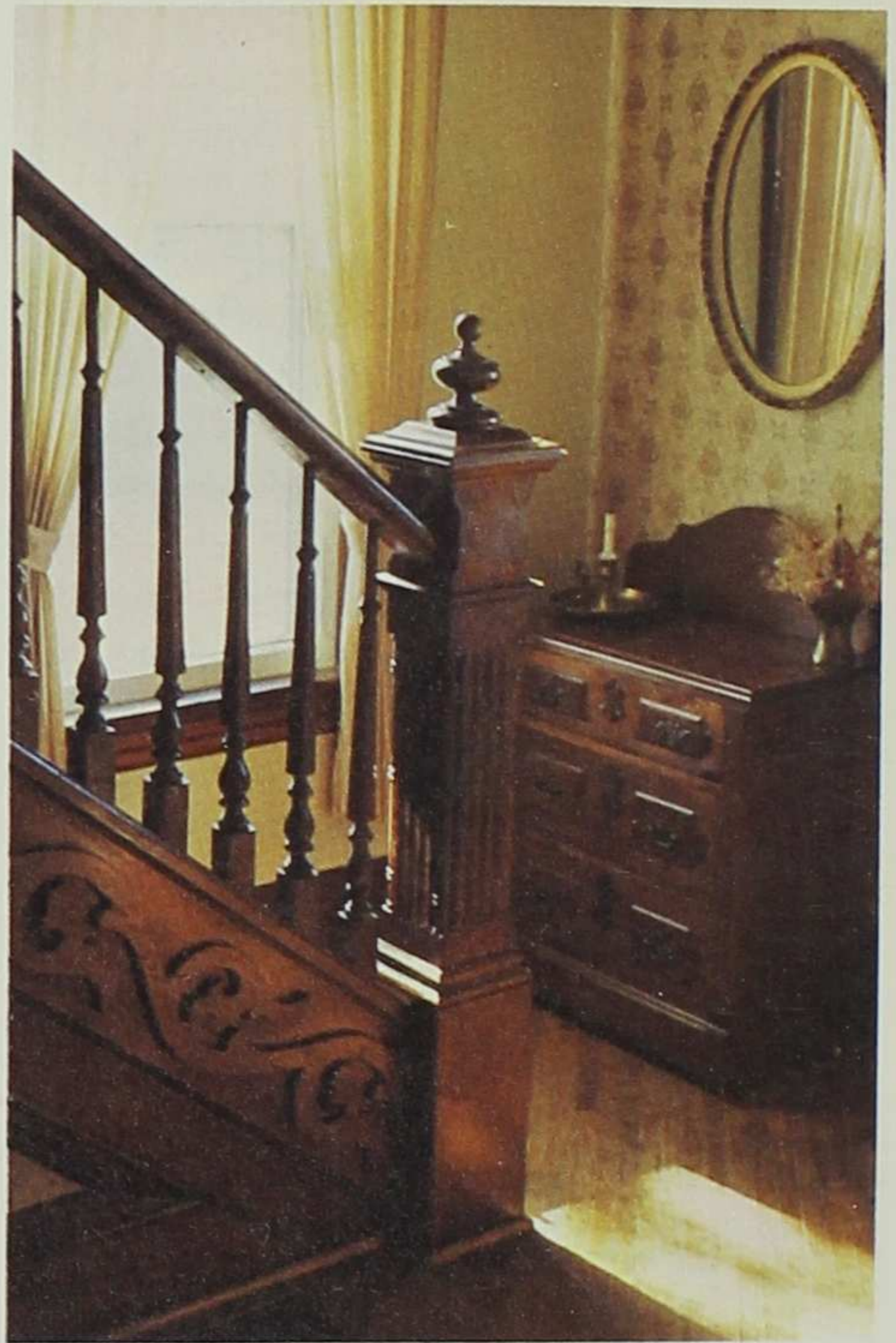
Located on an old post road (now a modern highway) near Springdale, Iowa, the Kenneth Mather house contains a beautiful millwork newel post and stair decoration. The scrollwork on the side of the stairs (called “stair brackets”) may be found in both the 1892 and 1904 Disbrow & Company catalogues.
