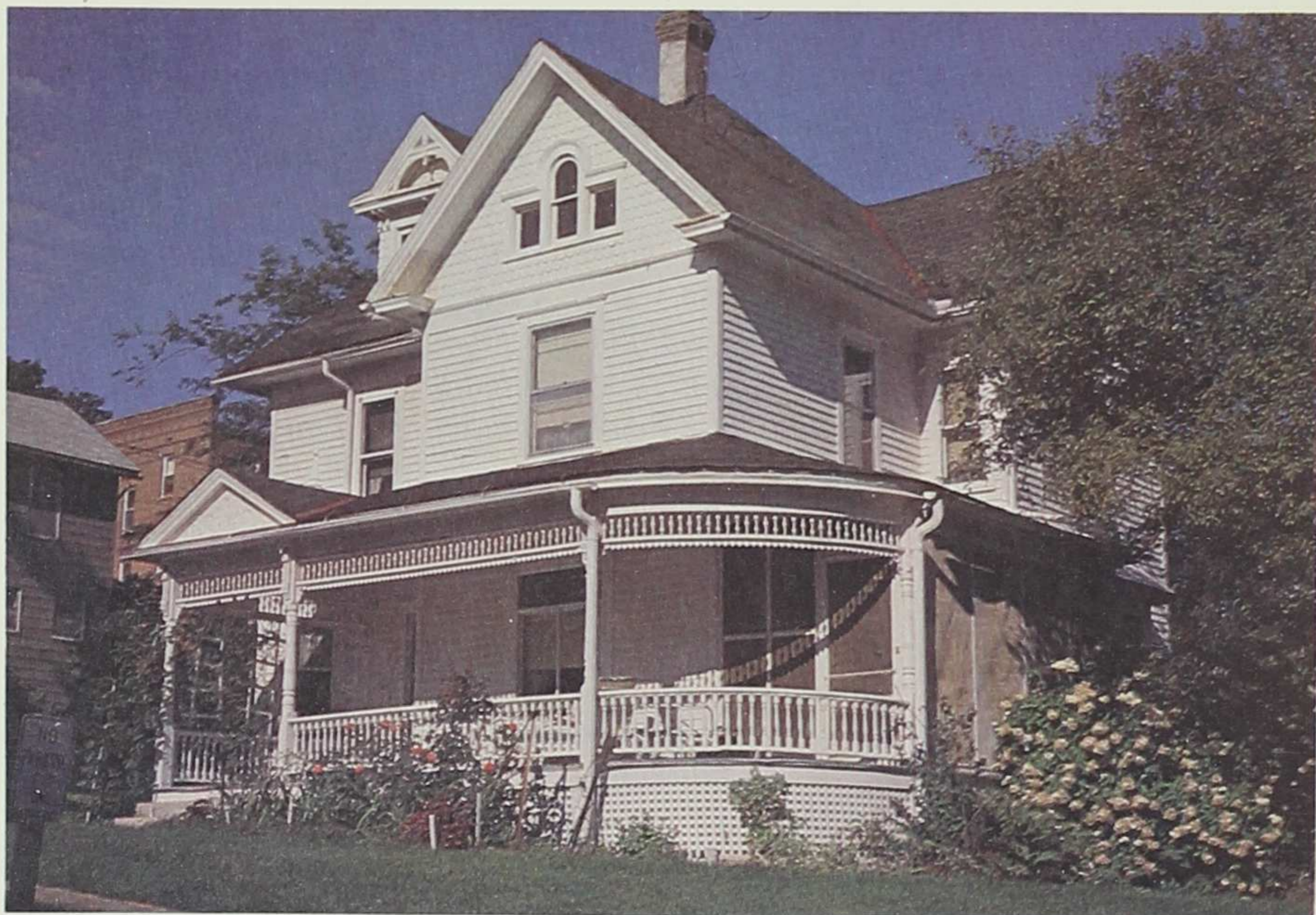
A porch extending around two sides of the house at the C. E. Gillette home in Mt. Vernon, Iowa.
