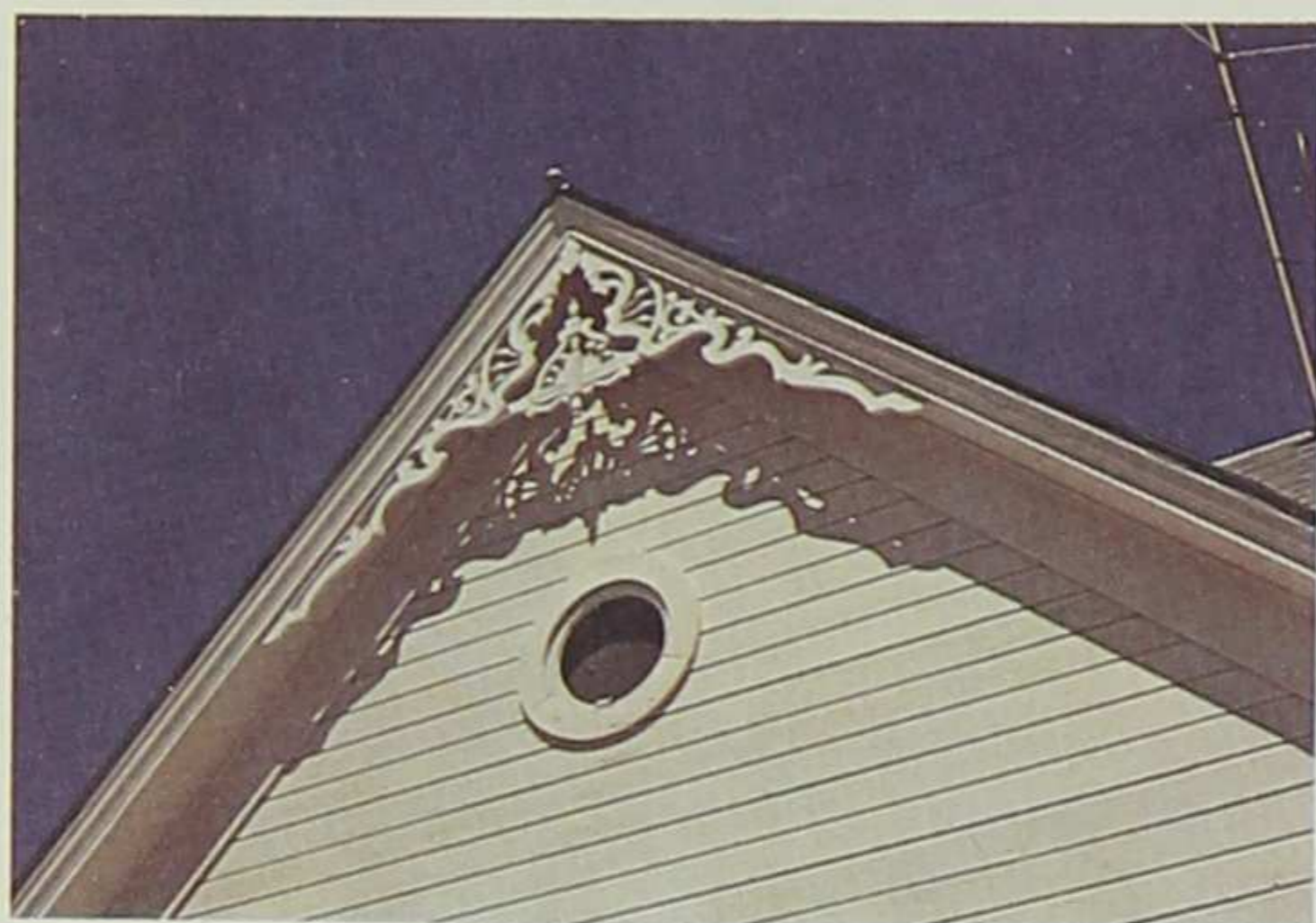
Gable finish from a house in Boulder, Montana, similar to an adjustable gable ornament shown in the 1909 Disbrow catalogue. Many of the Disbrow & Company's products were shipped to western states.
