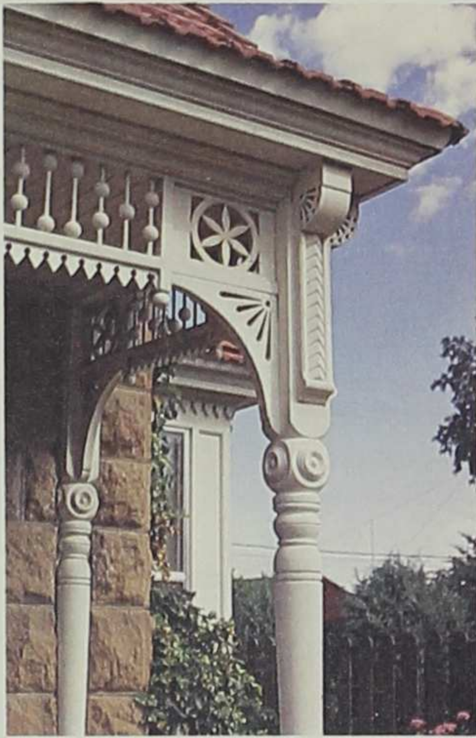
An ornate millwork porch detail from Blackfoot, Idaho.
