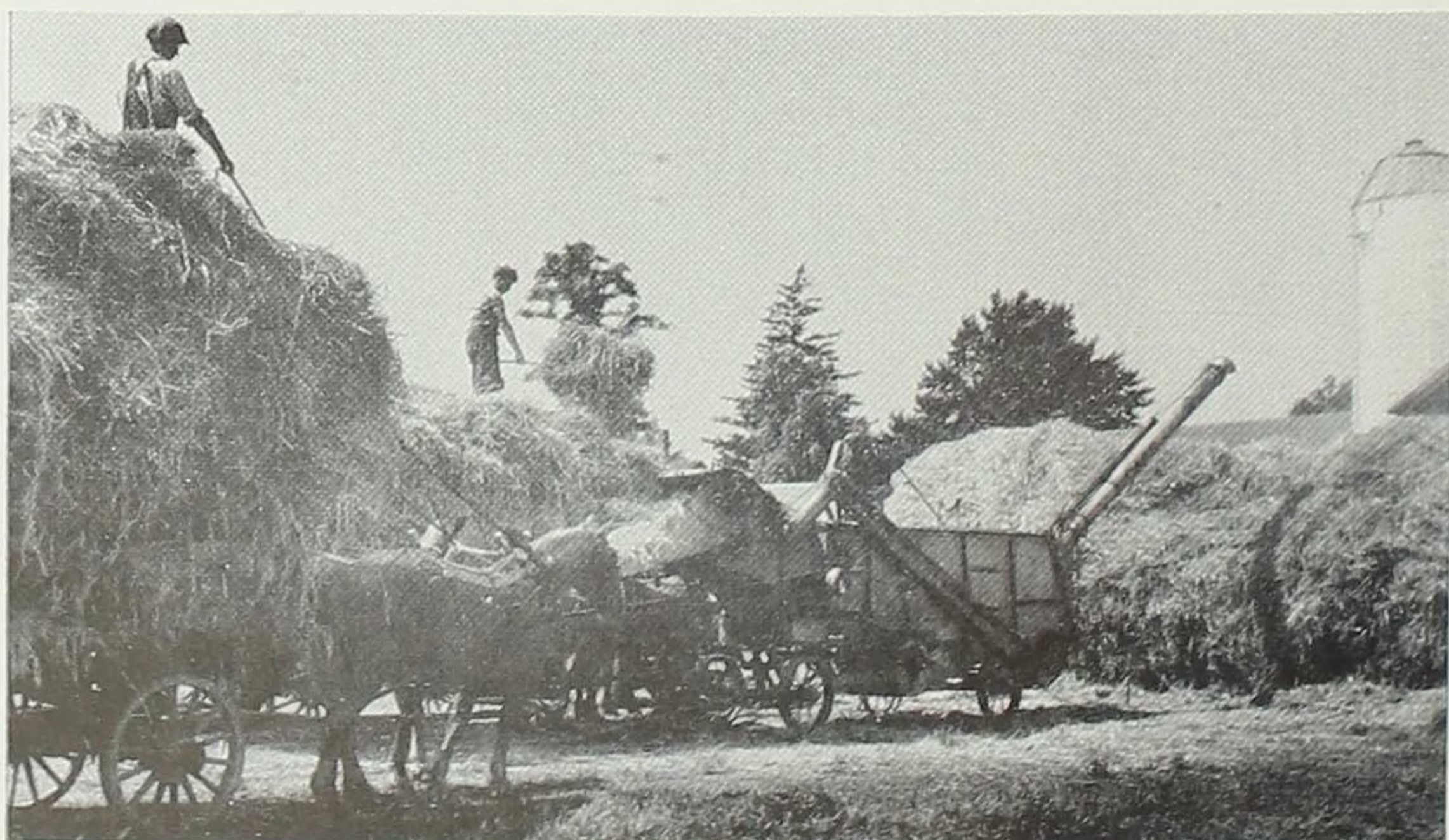
Thresher equipped with self-feed, wind stacker, and grain weigher.
