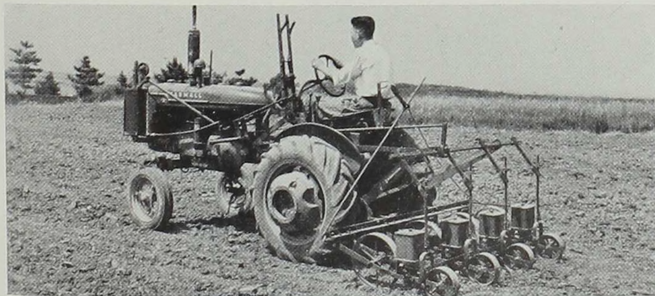
Direct connected four-row tractor garden drill.
