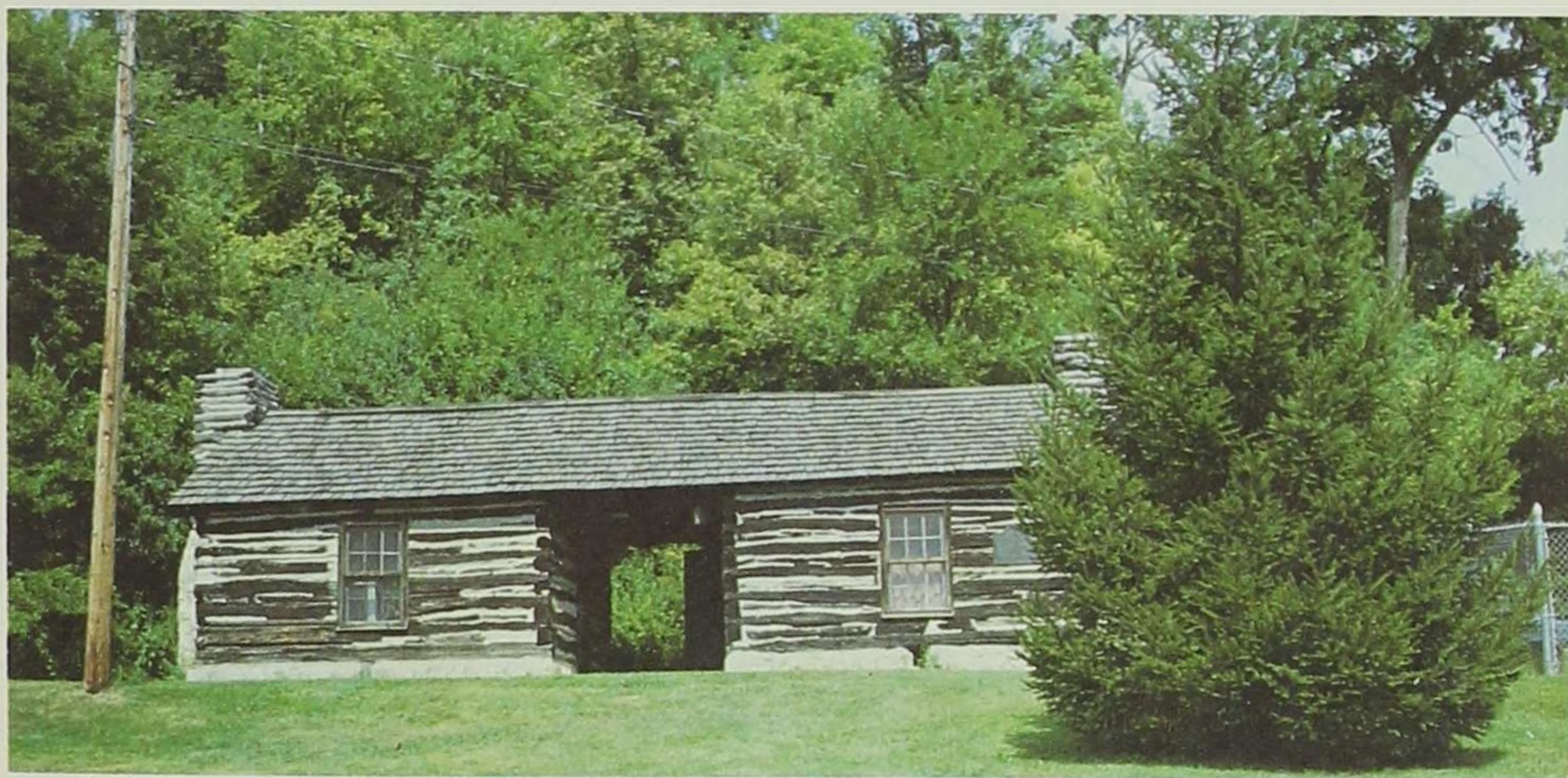
The William Newman cabin, of the dog-trot variety, existed by 1833 and is now preserved in Eagle Point Park, Dubuque. A dog-trot cabin was simply two single cabins joined together by a continuous roof, creating a breeze-way between them.
