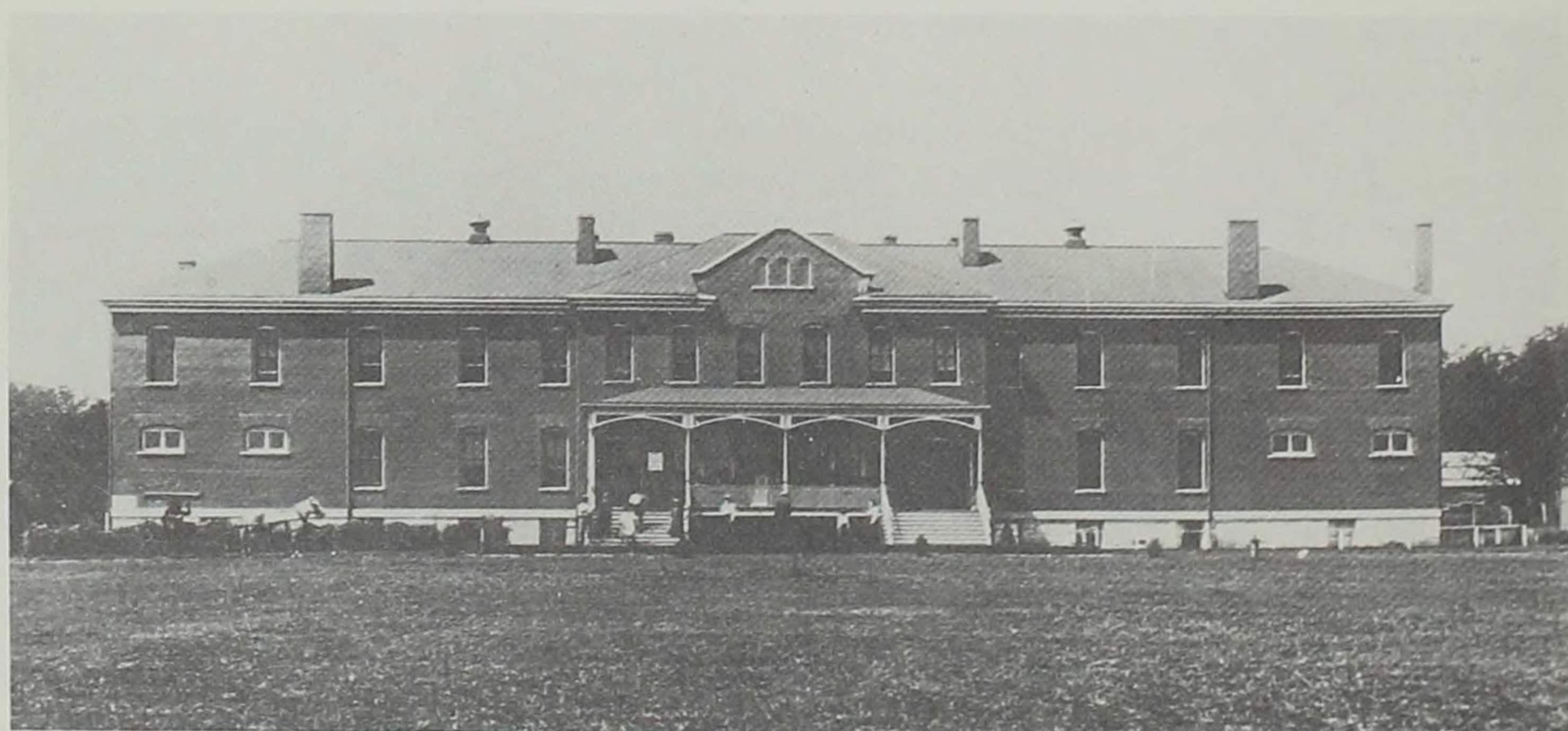
The Toledo Indian Training School, founded by Horace Rebok. Built at government expense, the building was used as a sanatorium after the failure of the school to attract Mesquakie children.
