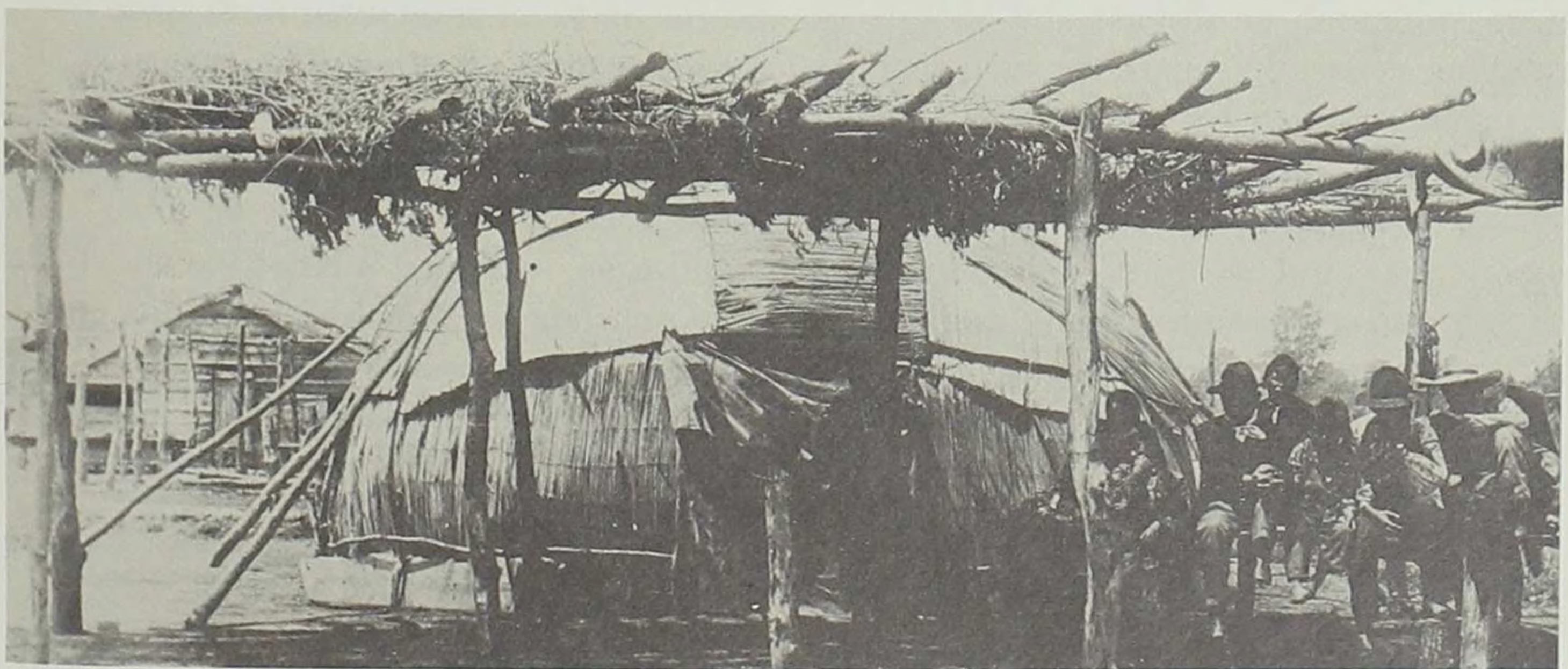
A summer shade which provided relief from the sun and usually was built adjacent to a wikiup. In the background to the left is a gable-roofed wikiup.
