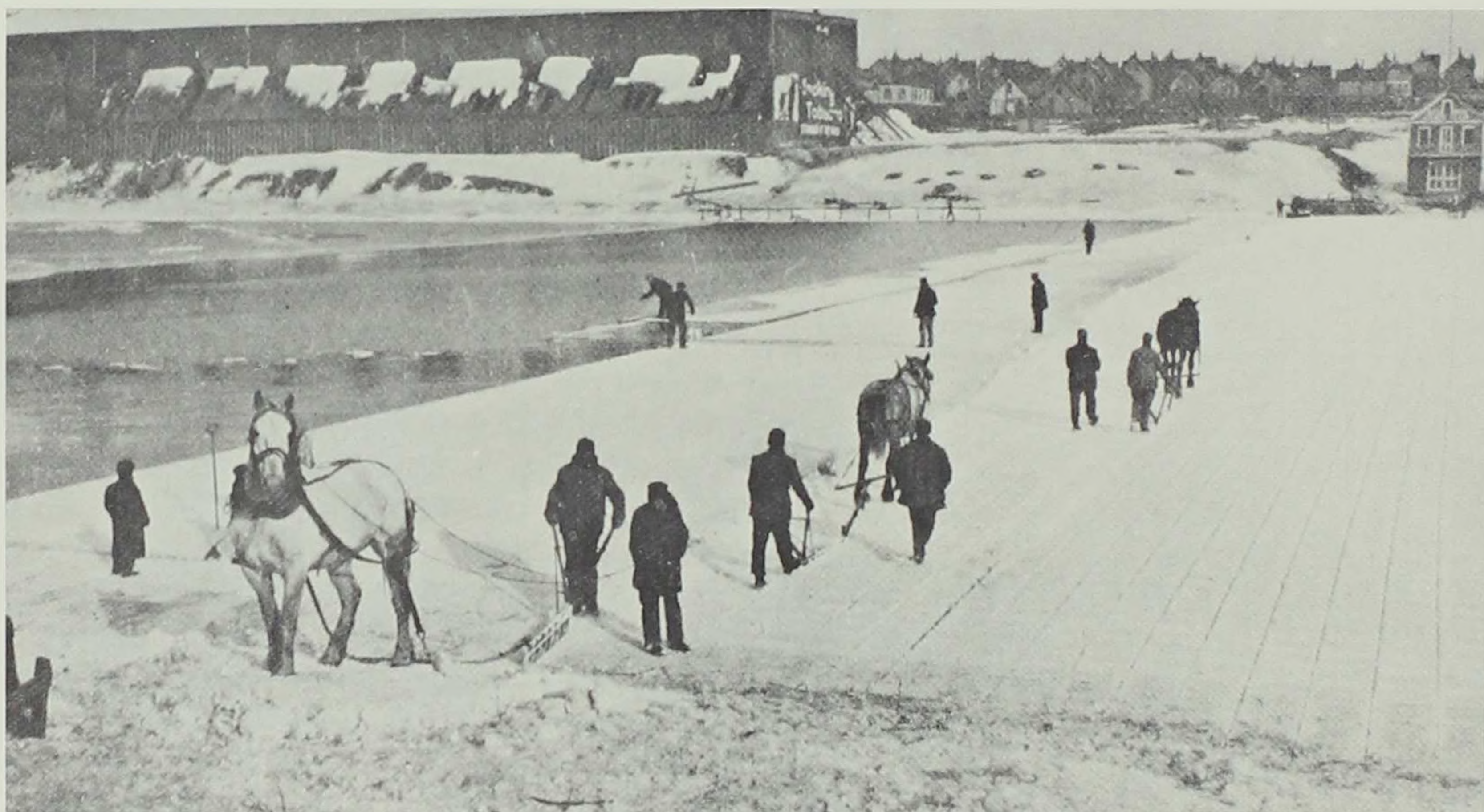
The ice harvest begins: surveyors have marked boundary lines and now horse-drawn ice cutters trace a grid pattern on the river's frozen surface. Deep cutters and ice plows will follow. (courtesy Cedar Falls Historical Society)
