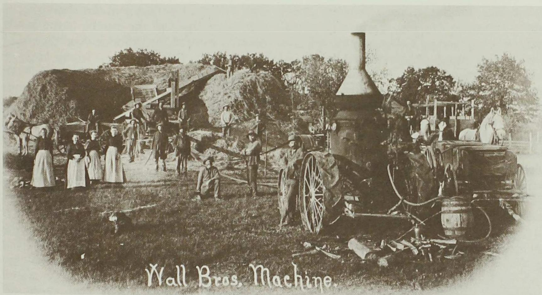
*The traction engine pictured in this threshing scene has an upright boiler — odd in appearance, but a common sight around the turn of the century. The engine appears to have chain drive. (SHSI)*
