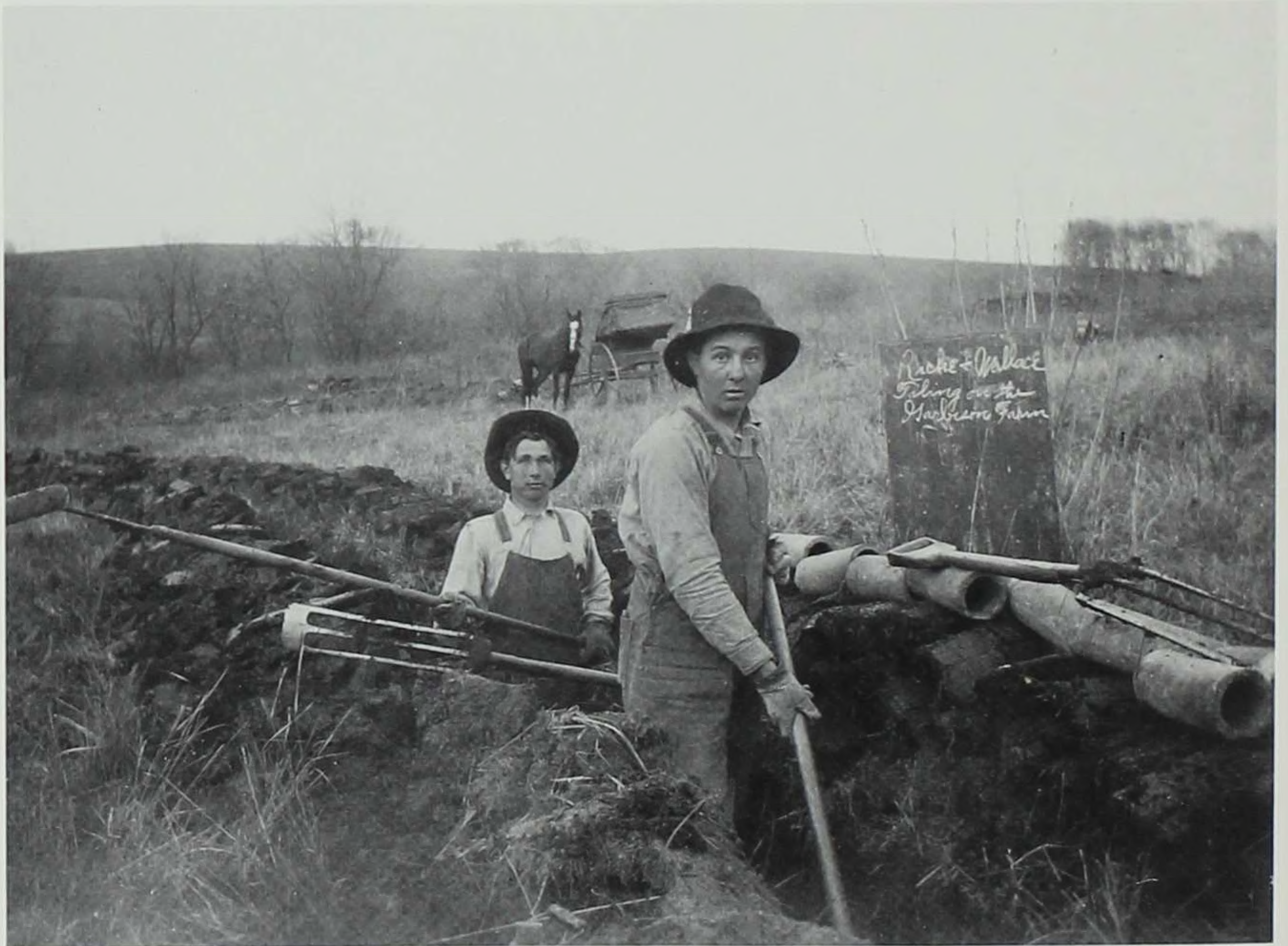
"Thur 4 May 1911 Alva Riche & Russell Wallace tiling on my place. Darko 60 counts." Note the clay drainage tiles and tools lying above the ditch. The phrase "Darko 60 counts" suggests that Garbison exposed the glass plate negative to sixty counts of light when he printed the image on "Darko" brand printing-out paper.
