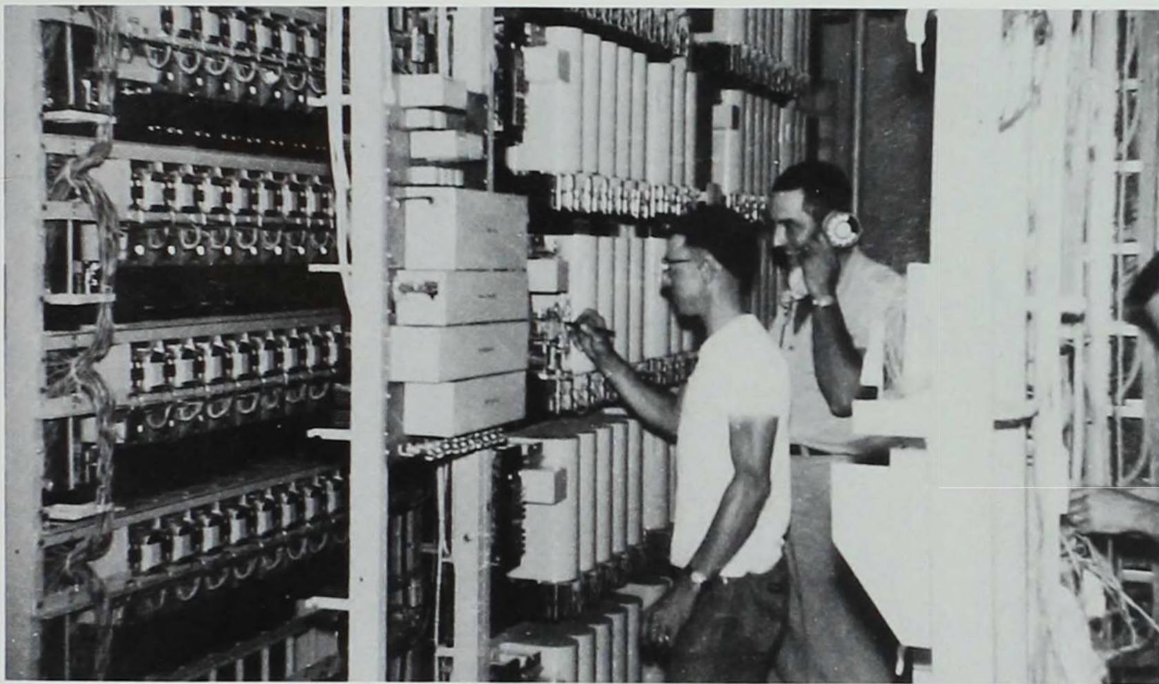
Equipment for the dial phone system in Strawberry Point in 1956 is checked over by Leland Carpenter and Robert Homewood. As dial systems were implemented, switchboard operators were phased out.
