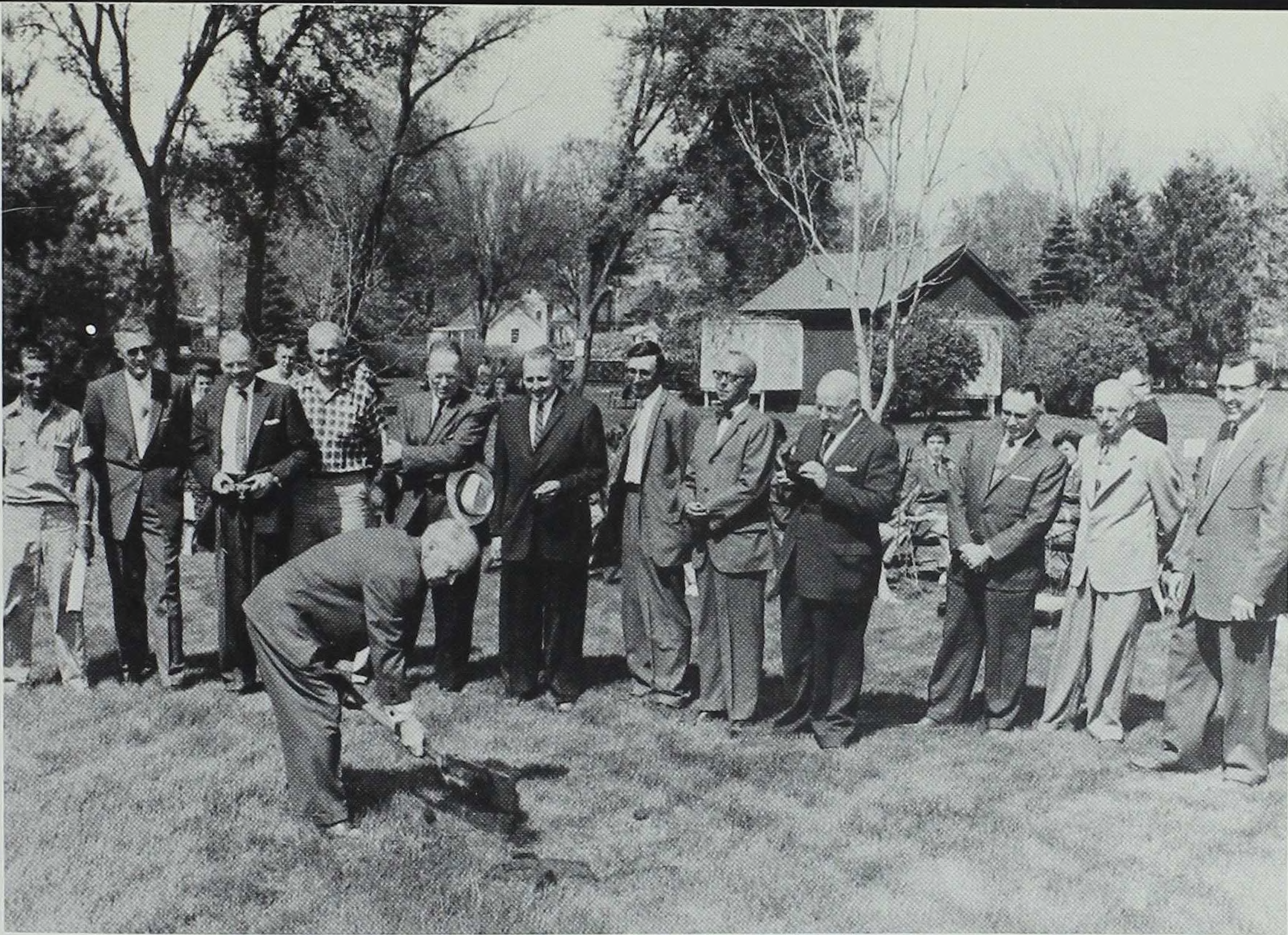
Foundation president William B. Anderson breaks ground for the library-museum on May 4, 1959. The birthplace cottage is the small white building in the distance. Behind Anderson (from left): William Smith, construction firm superintendent; L. D. Vickers, administrative assistant to Fred Maytag; Fred Maytag, trustee; William Weber, of Weber Stone in Stone City; John M. Henry, trustee; Paul M. Jensen, vice-president of Viggo M. Jensen construction company; Floyd Fawcett, R. B. Figge, Ralph Evans, L. C. Rummells, and John Thompson, all trustees; and Rev. L. E. Bauman, who gave the invocation.
