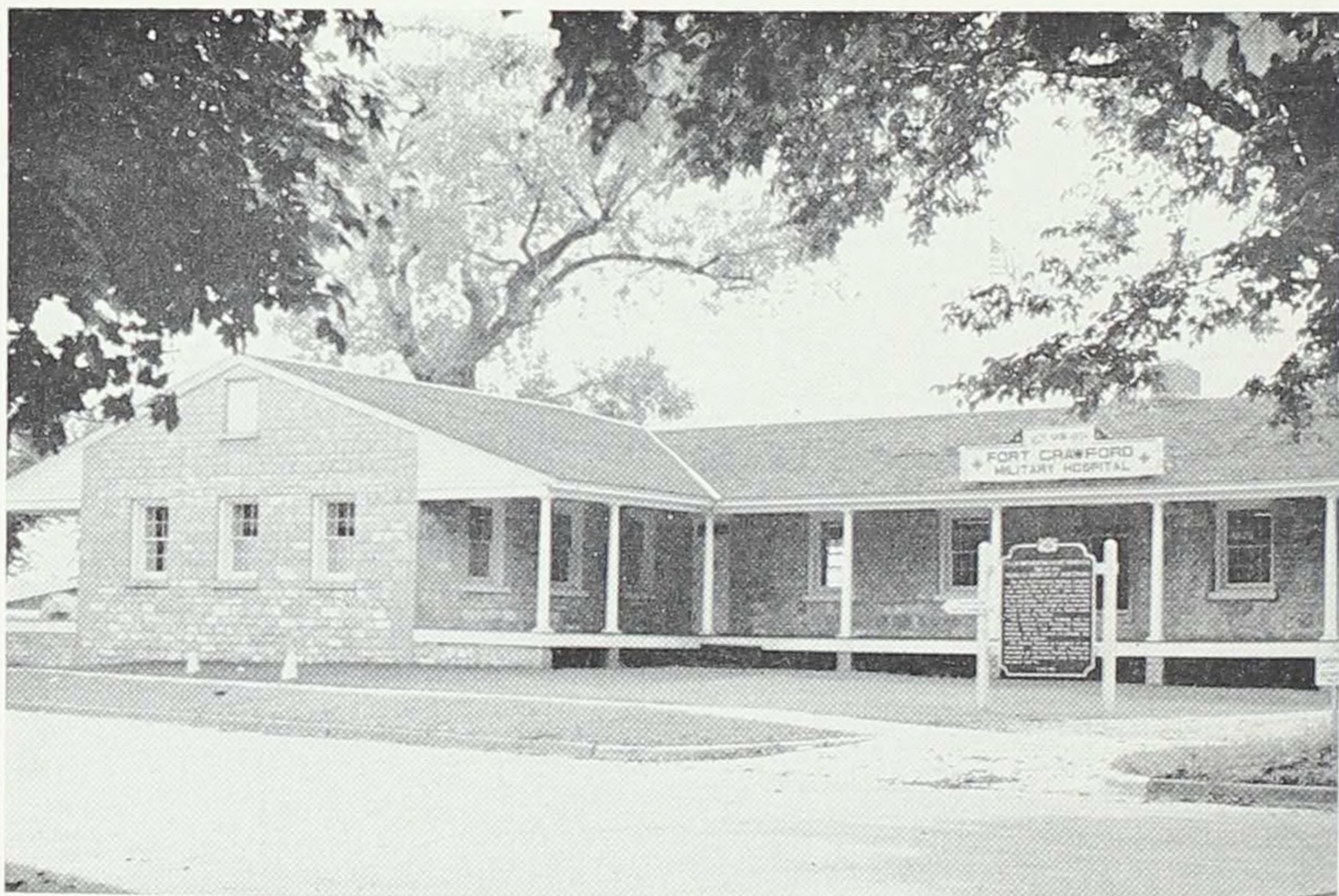
Restoration of Second Fort Crawford Hospital. Houses the Museum of Medical Progress Established by the State Medical Society of Wisconsin
