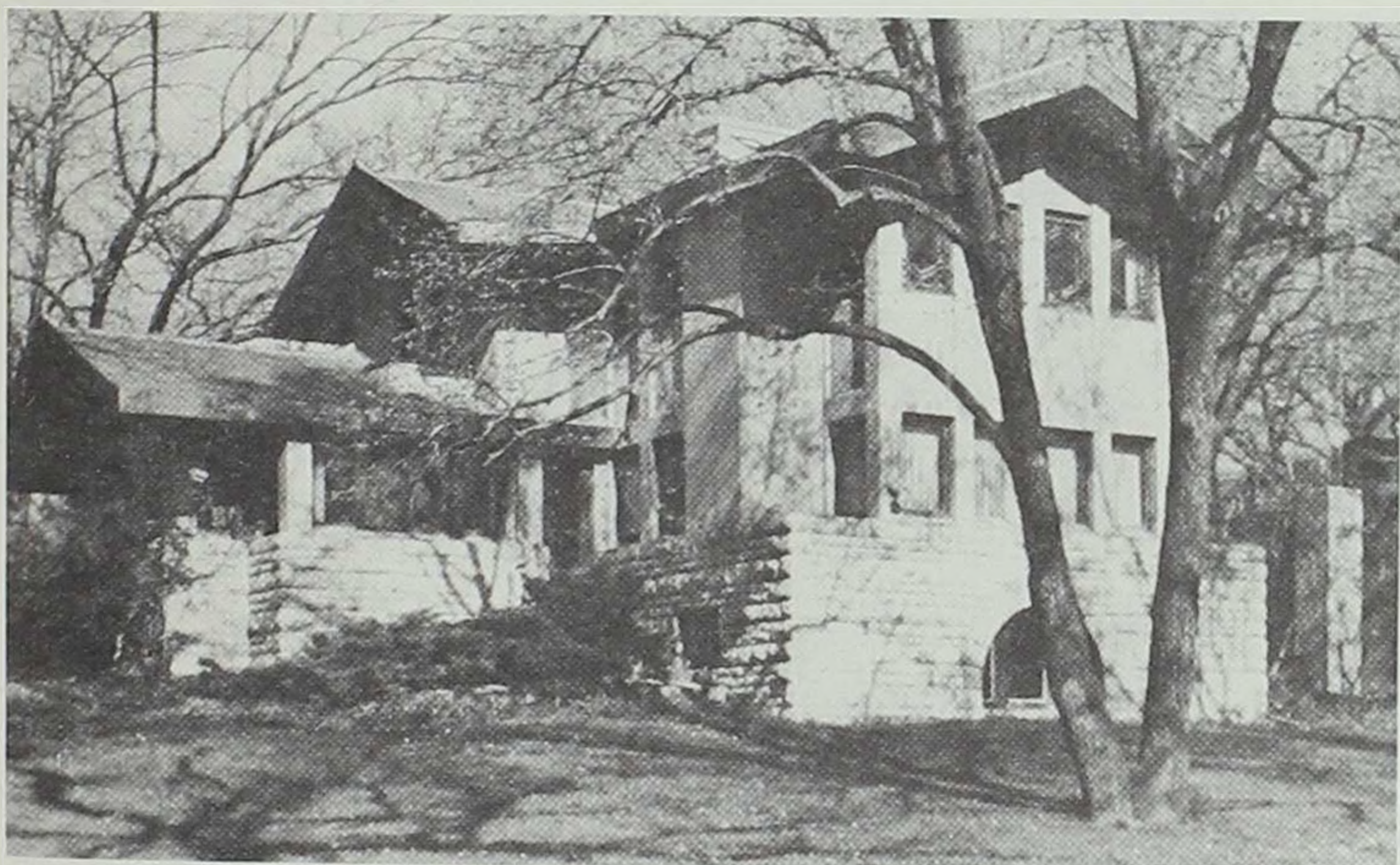
The Page house (1912) is characterized by a high, tight design, with walls built of an exposed reinforced concrete framework that adds to the ornamental effect of the house. The roof is gabled, with projecting flared eaves, and rough ashlar distinguishes the ground level.
