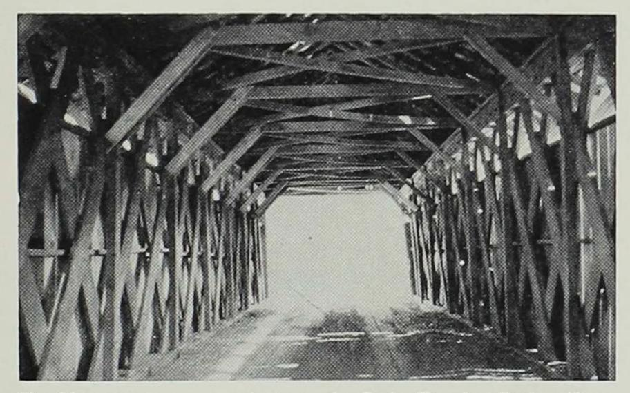
The Town lattice truss is shown in the Cutler-Donahoe Bridge. Trunnell pins, rather than bolts, were used in what remains of the original structure.
