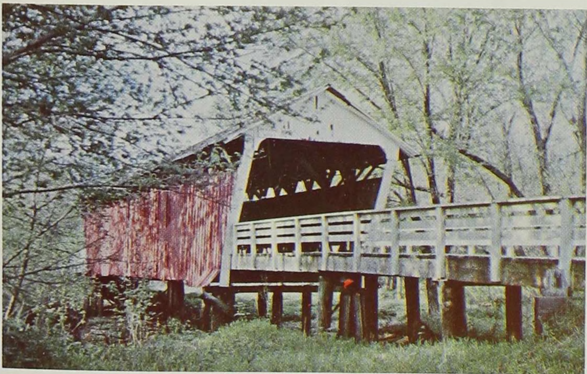
Cutler-Donahoe Bridge — Madison County.
