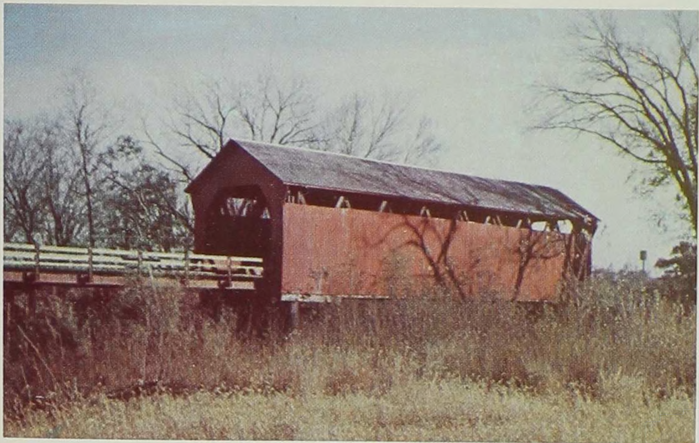
Hammond Covered Bridge — Marion County. (Photograph by Sperry)
