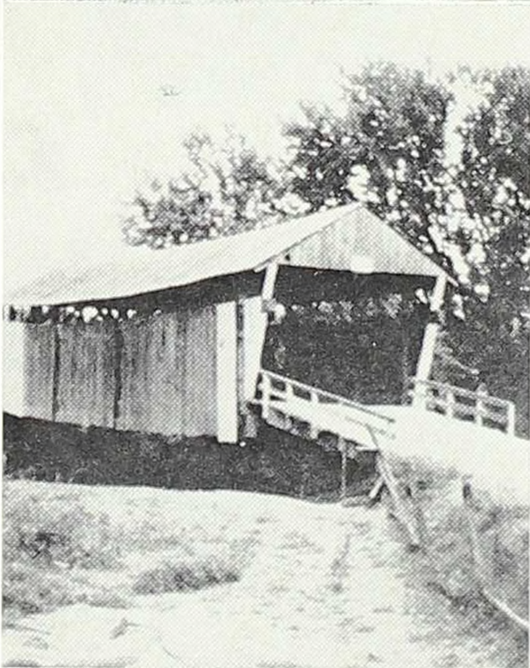
(Above) Clayton County's Mederville Covered Bridge, soaring 75-80 feet in the air, had an incredible length of 255 feet without a center supporting pier. It was the longest single span bridge in Iowa and one of the highest in the country. (Photograph from Les Swanson.)
