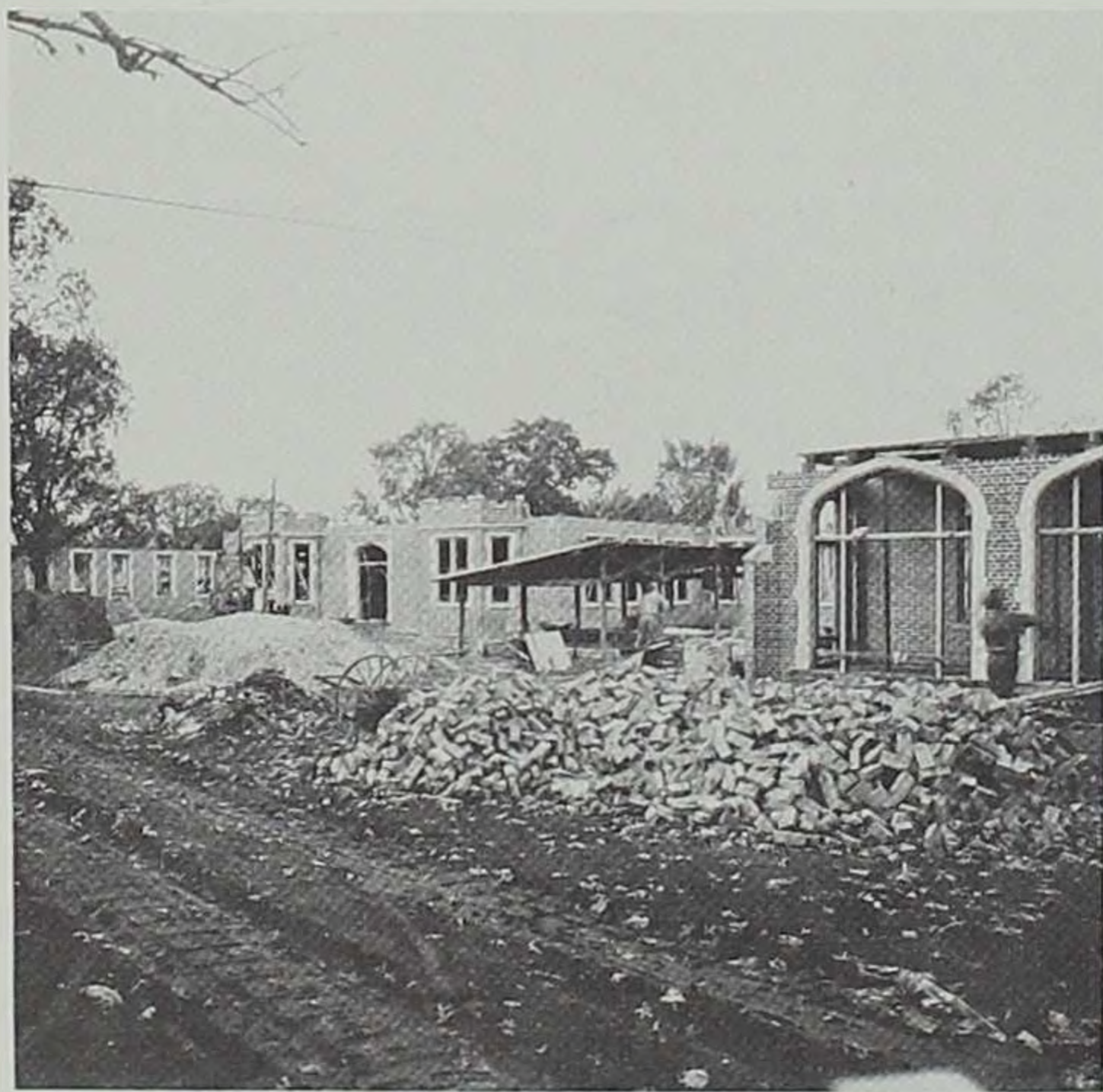
A 1920 view of the Hospital under construction.
