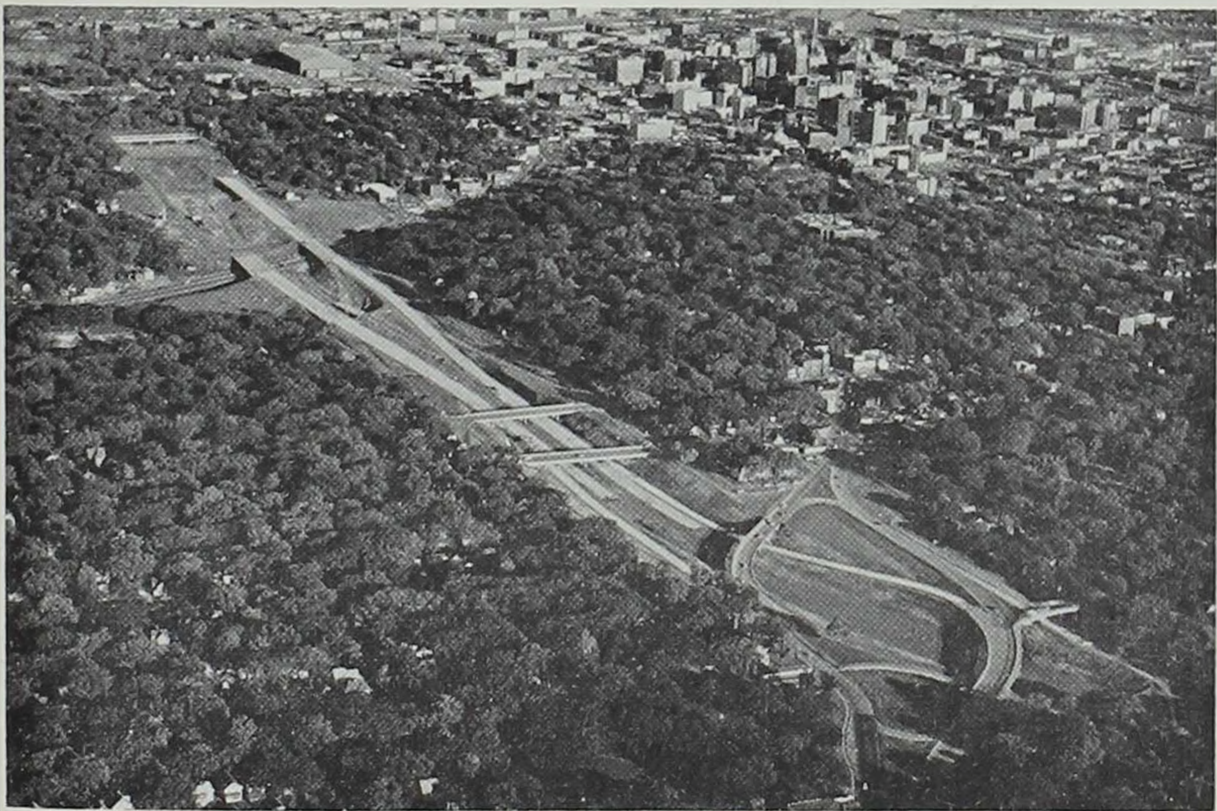
The $57 million Des Moines Freeway is part of the Iowa Interstate system. It will not only provide a connecting link through Des Moines to the Interstate routes skirting the city, but will also relieve heavy congesting traffic on local streets.
