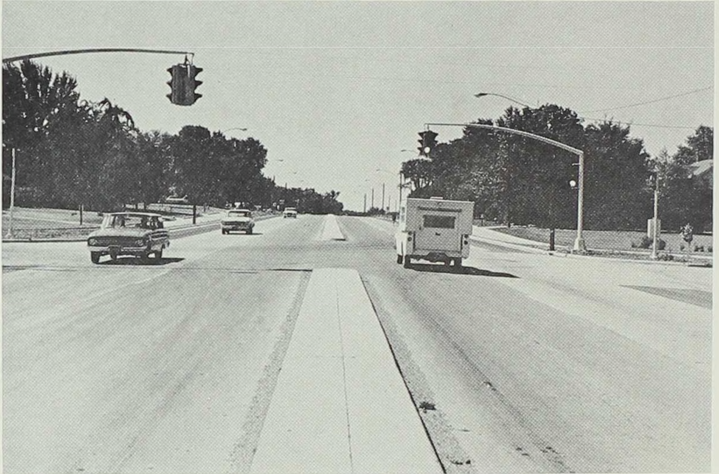
This is a primary municipal extension at the north edge of Ottumwa on U.S. 63. This four-lane, divided thoroughfare, provides an attractive entrance to the city and replaces an old two-lane road.
