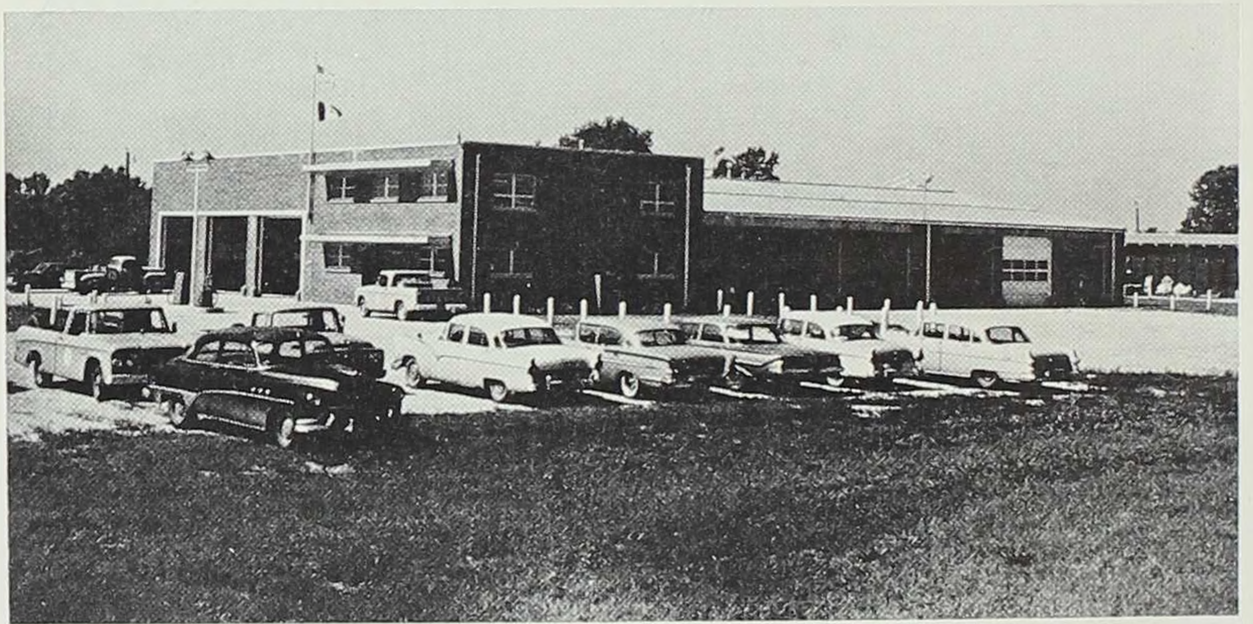
New highway maintenance garage on Iowa 192 south of Council Bluffs.
