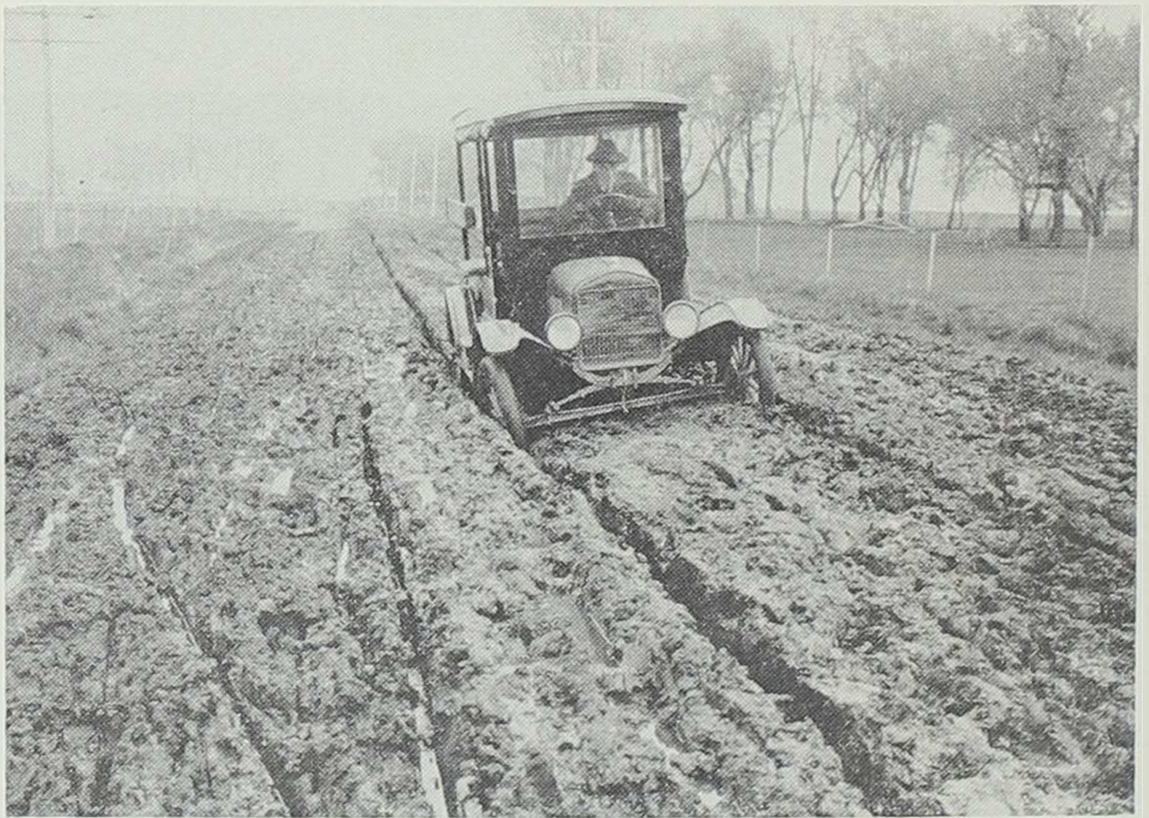
The famous Lincoln Highway between Ames and Nevada in 1918. The driver of the motor truck was not consoled by the knowledge that the road had a gravel surface. Unless properly drained a gravel road is no improvement over a dirt road. The Lincoln Highway was the most famous of the name roads that dotted the state and the country before the adoption in the 1920's of the system of numbering roads. The Lincoln Highway became U.S. Highway 30 and was entirely paved by 1928.
