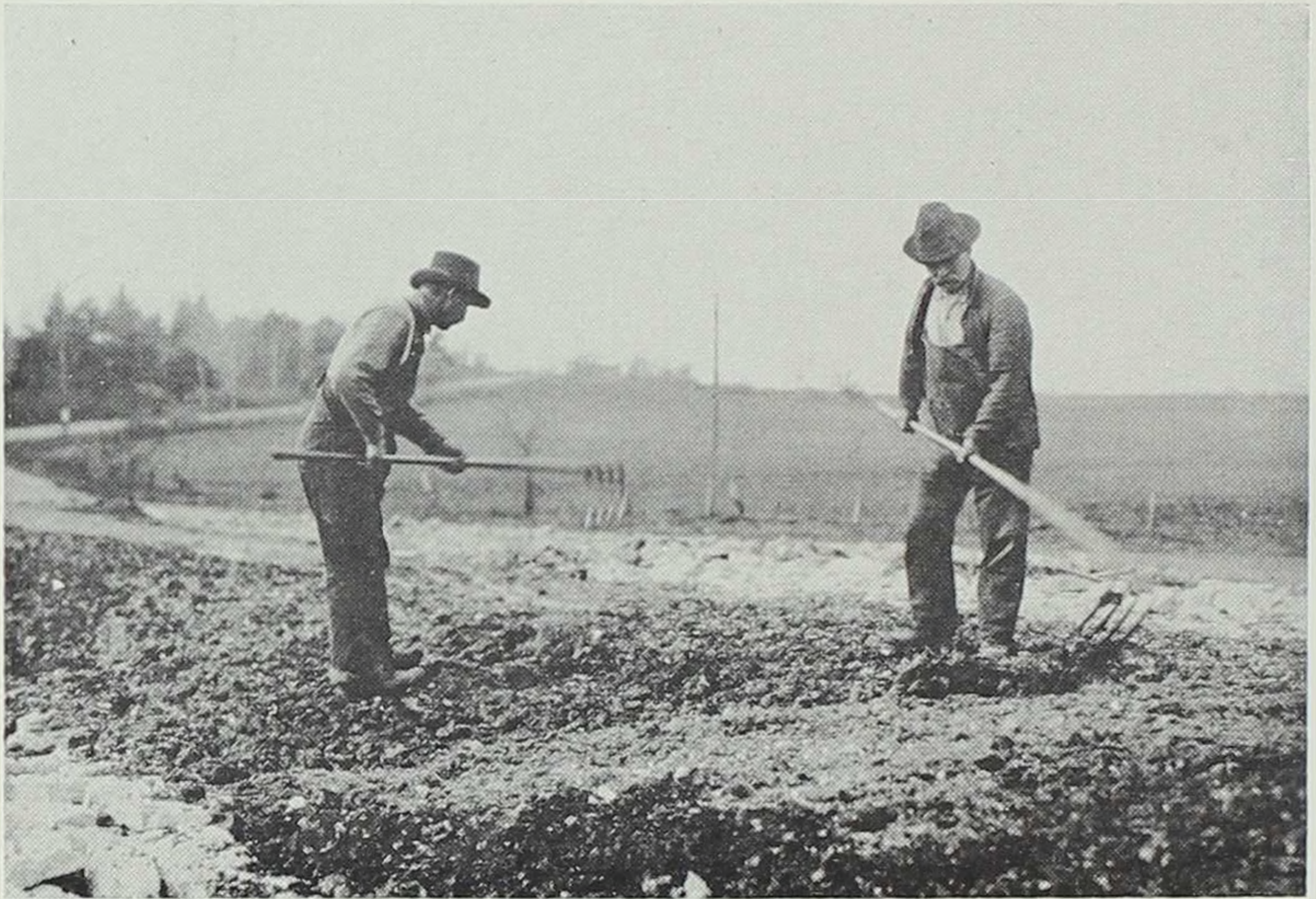
Road building tools and methods were still in a primitive stage of development in 1915, as indicated by these workmen on the Dubuque-Dyersville gravel road construction project. This was Iowa's second road to receive federal aid.
