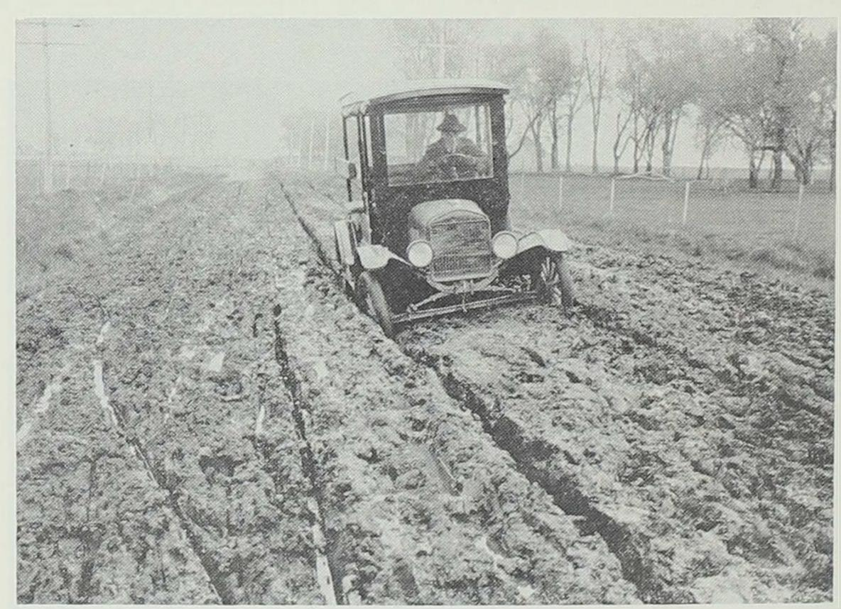
The famous Lincoln Highway between Ames and Nevada in 1918. The driver of the motor truck was not consoled by the knowledge that the road had a gravel surface. Unless properly drained a gravel road is no improvement over a dirt road. The Lincoln Highway was the most famous of the name roads that dotted the state and the country before the adoption in the 1920's of the system of numbering roads. The Lincoln Highway became U.S. Highway 30 and was entirely paved by 1928.
