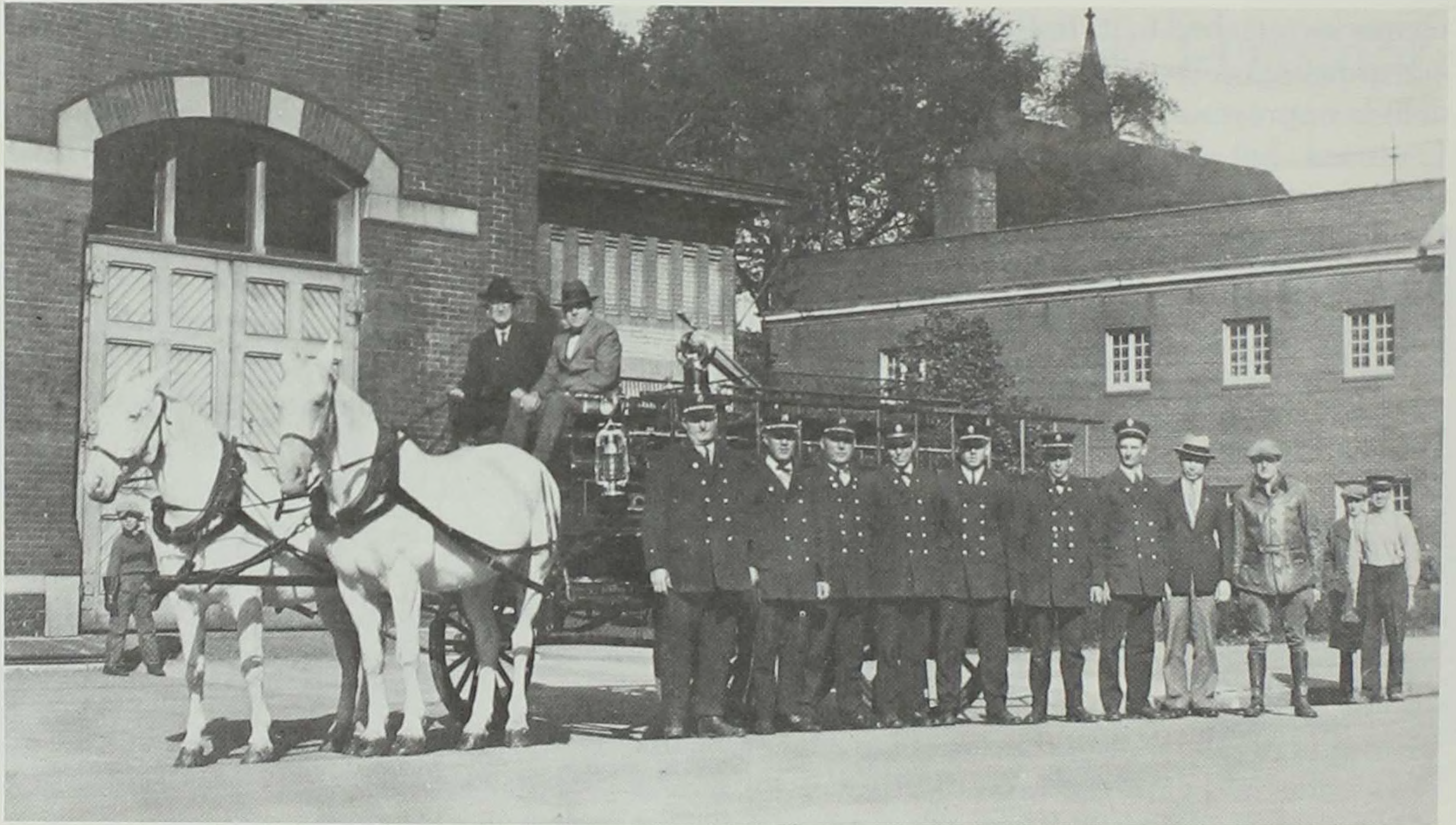
Fire station in the City Hall, c. 1920. The author can be seen beneath the horse's head. The two gentlemen on the fire wagon are Mayor Jack Carroll and the author's father. (courtesy Carl B. Cone)
