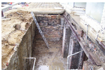
Underground Sidewalk Project
