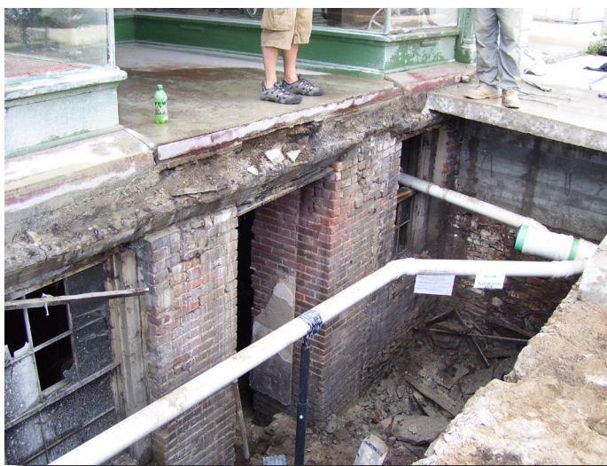
Underground Sidewalk Project
