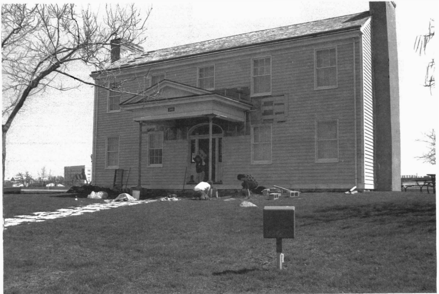
Fig 1 Excavations being conducted in the area of the porch at the 1833 Colonel Davenport House at the Rock Island Arsenal, Rock Island, Illinois.
