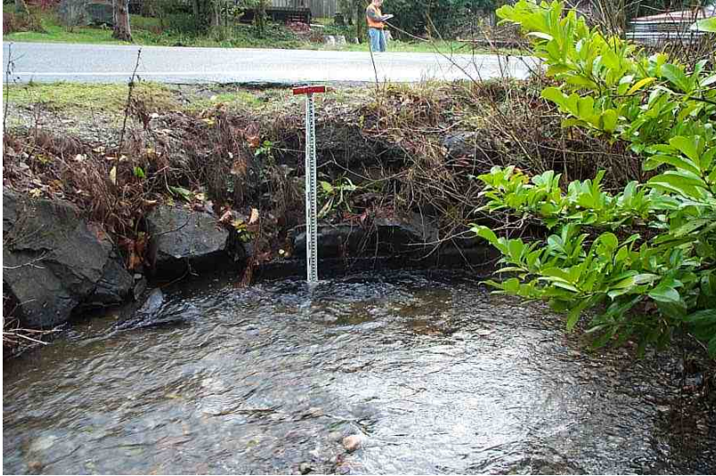
Before – 5 foot concrete box
