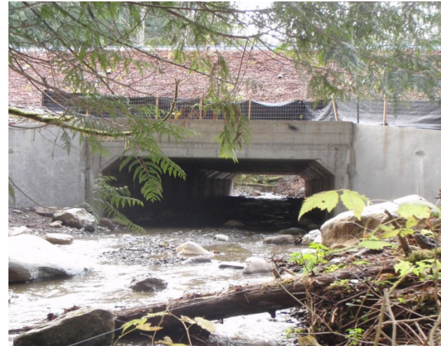
SR 112 Nelson Creek near Port Angeles
