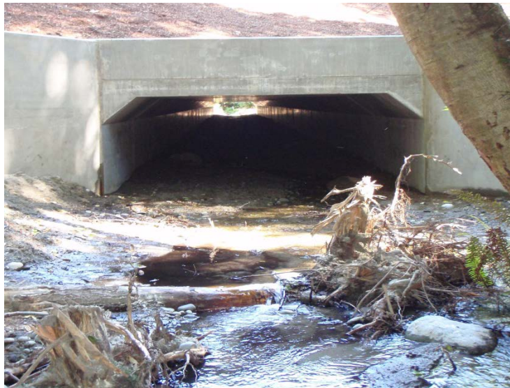
After – 12 foot 3-sided constructed in 2009
