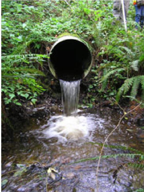
Before – 2.5 foot CMP with 2 foot drop
