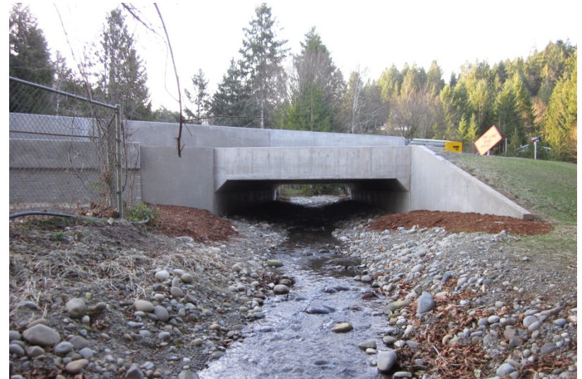
After – 20 foot 3-sided structure constructed in 2013
