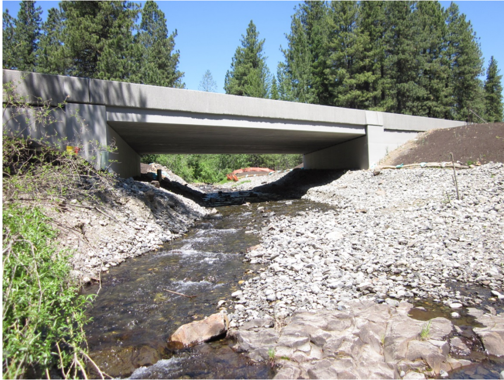
After – 65 foot bridge constructed in 2012
