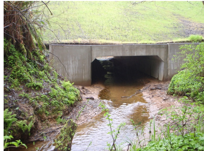
After – 16 foot Concrete Culvert constructed in 2009
