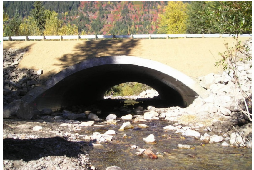
After – 37 ft arch constructed in 2006
