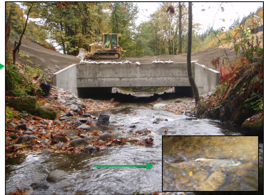
After – 34 foot bridge project completed in 2012
