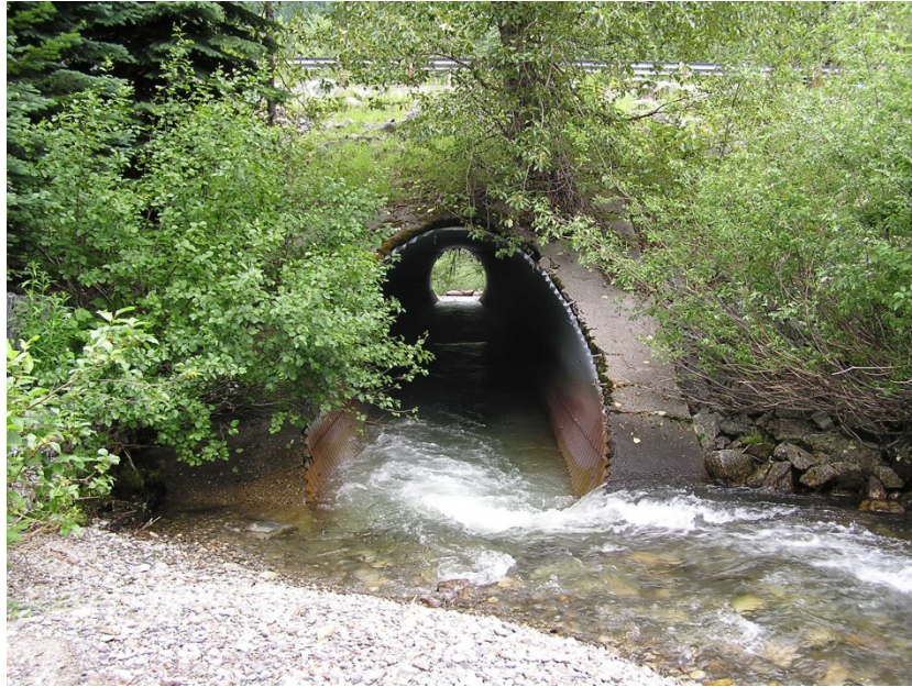
Before – 11 foot CMP was a velocity barrier
