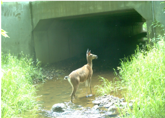
After – 16 foot Concrete Culvert constructed in 2009
