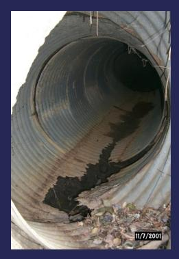
Piping: water runs outside the pipe causing void in road
