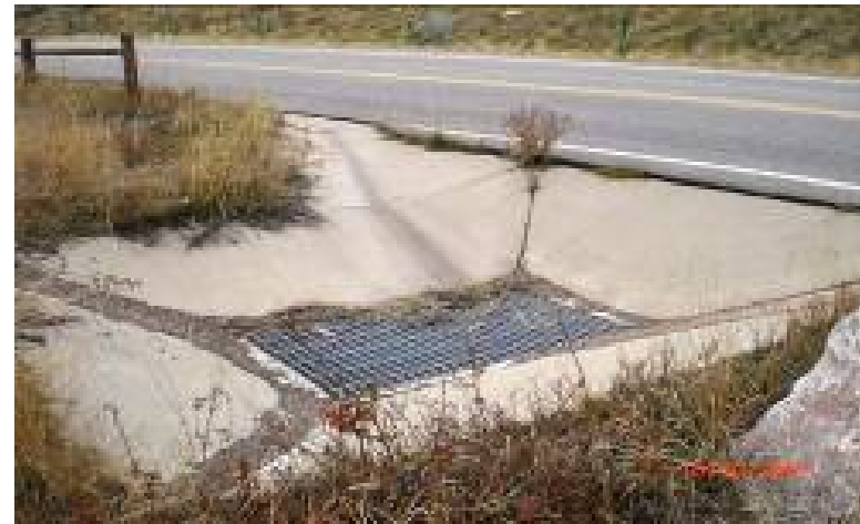
Type D Inlet (Closed Mesh)
