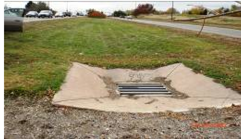
Type C Inlet (Standard)
