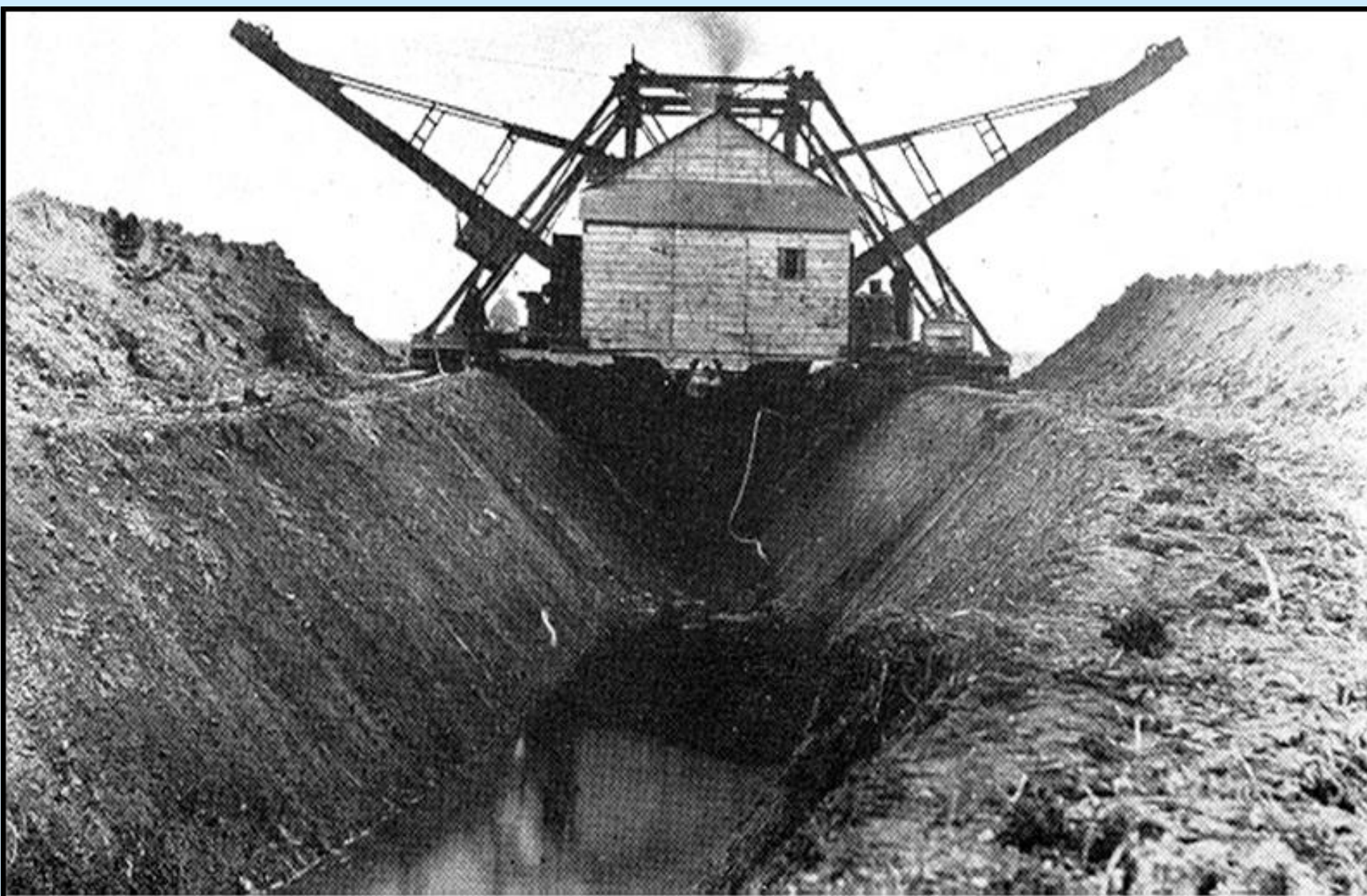
Excavating a large ditch using steam power, circa 1910.
