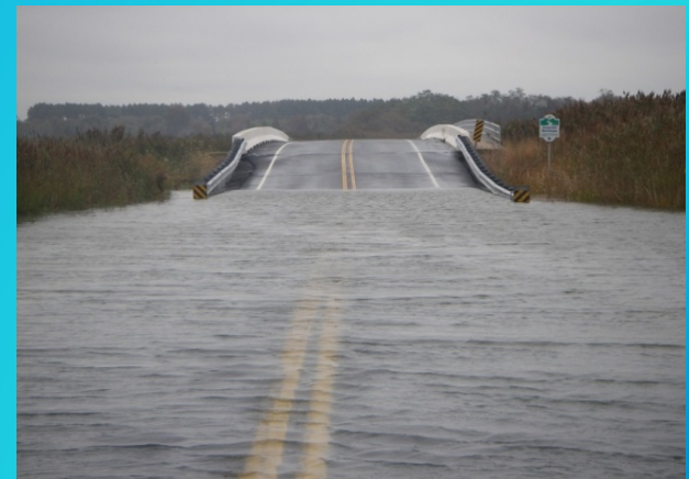
Daily Tidal Flooding – DE 9
