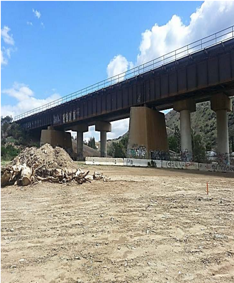
BNSF RR Bridge – view across left overbank
