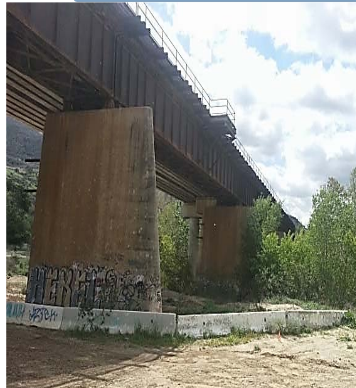
View downstream along pier columns
