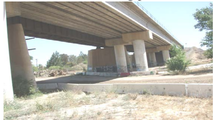
View across right overbank
