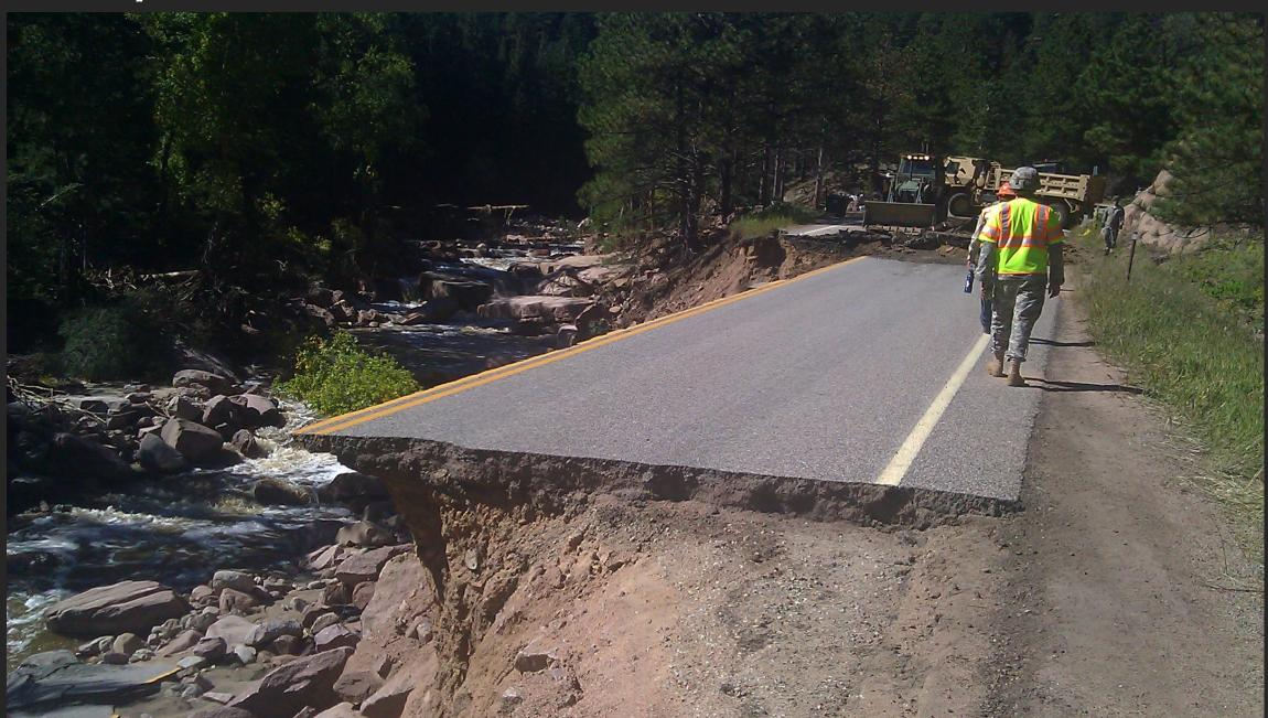
1. State and Federal highway bridges survived, though bridge approaches failed
