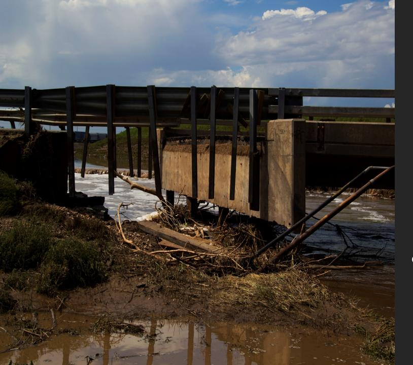
Washed Out Bridge Approaches on Highway Bridges
