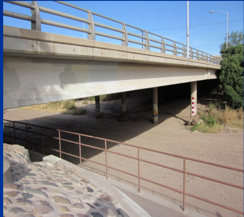
Congress Street Bridge on Santa Cruz River
