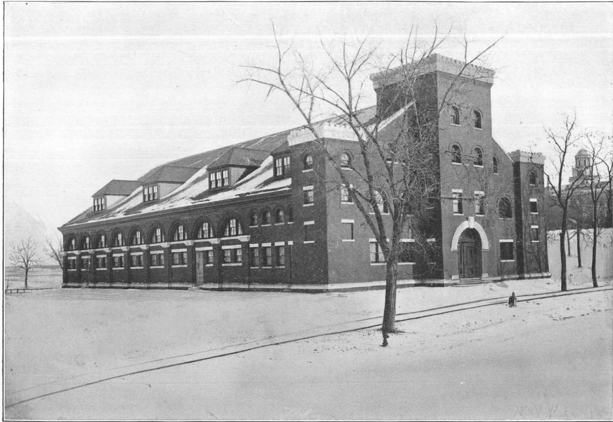
THE ARMORY AND ATHLETIC PAVILION
